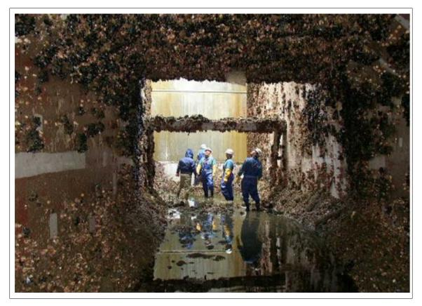
Figure 4.3 Mussel infestation in a main cooling water culvert (drained for maintenance) (By permission of KEMA)
