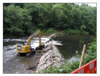
Figure C.7 Prestolee Mill weir removal
