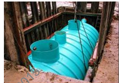
Example of a full retention separator during installation.
