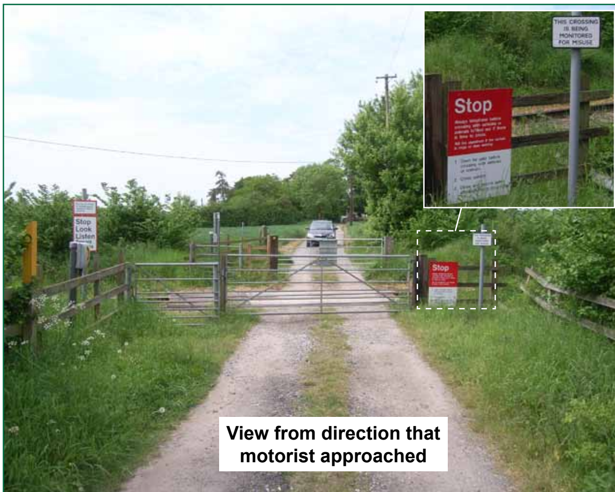
Figure 4: The approach to Lindridge Farm user worked crossing and its signage
