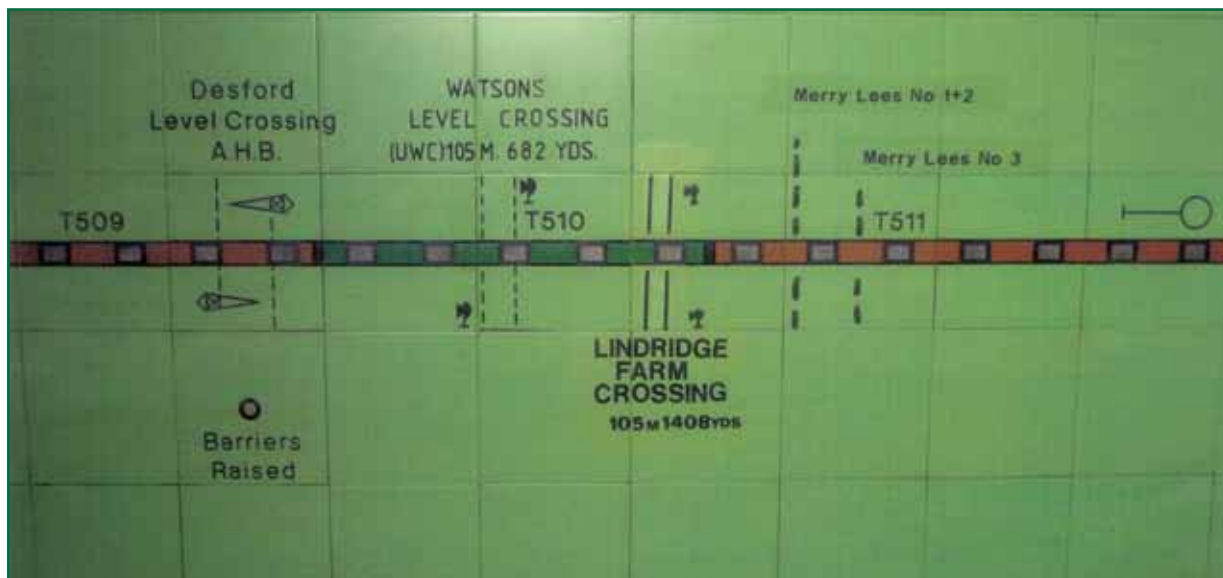
Figure 19: The signaller's panel at Leicester signal box with the Merry Lees user worked crossings incorrectly marked up on track section T511
