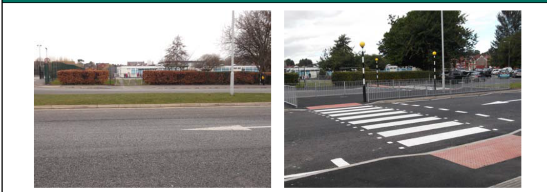
Figure 4.5 Before and after the installation of a double zebra crossing at St John Plessington College in Wirral, identified by students doing a School Route Audit as key to encouraging walking to school (Images courtesy of Living Streets)
