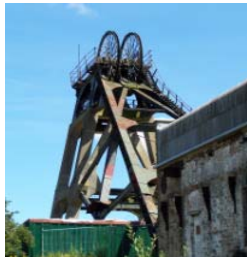
Former colliery at Pleasley, Nottinghamshire
