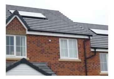
Sustainability approaches and features incorporated into the Code Level 3 units include solar thermal water heating, low flow rate sanitary ware, the use of water butts to collect rainwater, the design of all homes to Lifetime Homes, the use of more environmentally benign materials, higher levels of insulation, low energy lighting, internal recycling bins.
