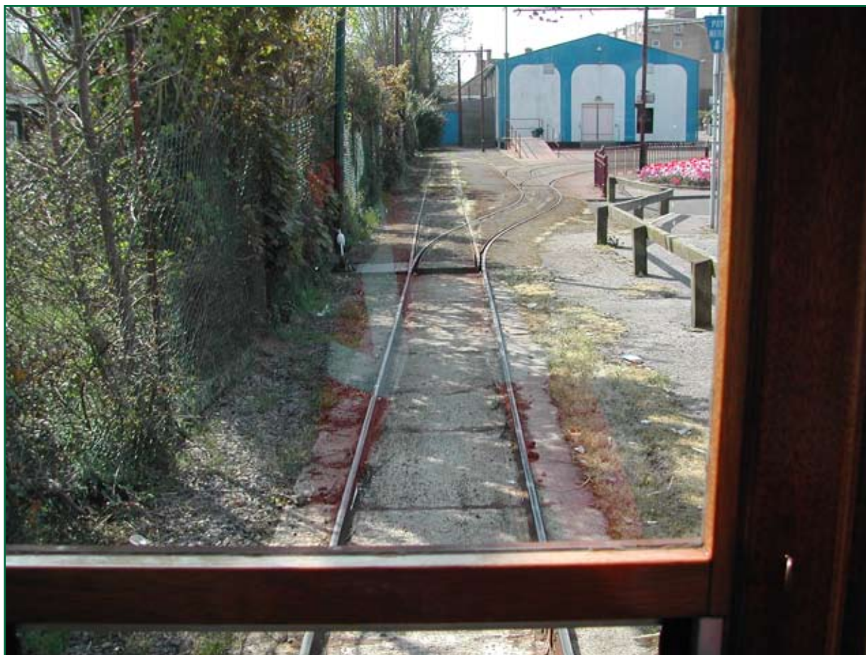
Figure 8: Driver's view approaching Seaton station
