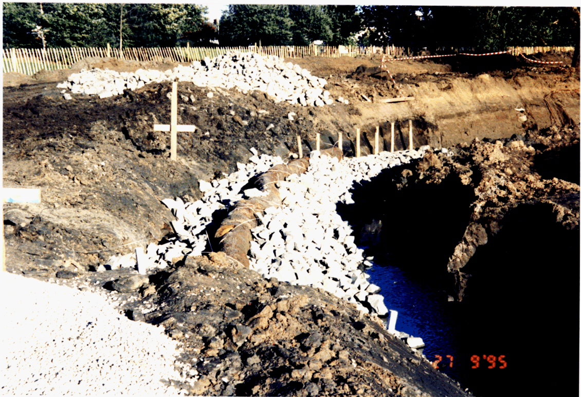
10. Log and geotextile during construction - logs wired over rock
