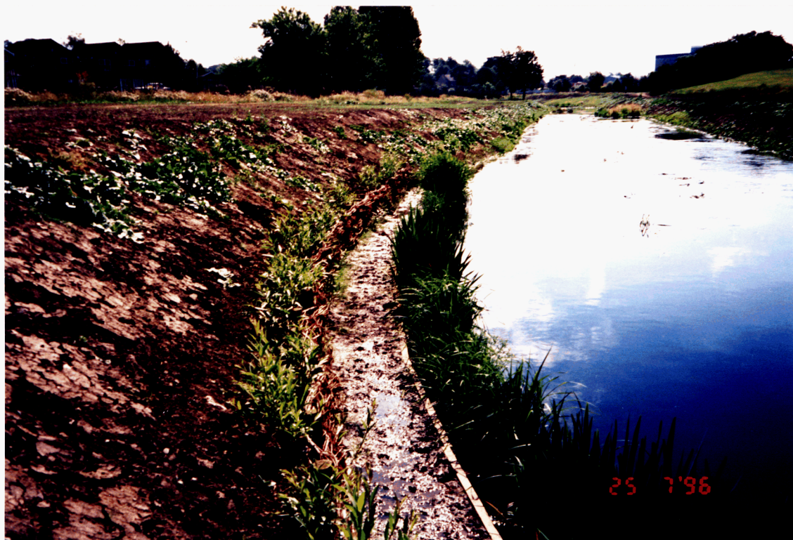
4. Entry spiling two months after installation
