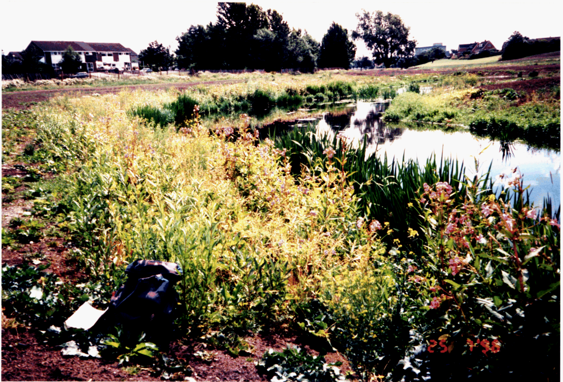
21. Willow mattress eight months after installation
