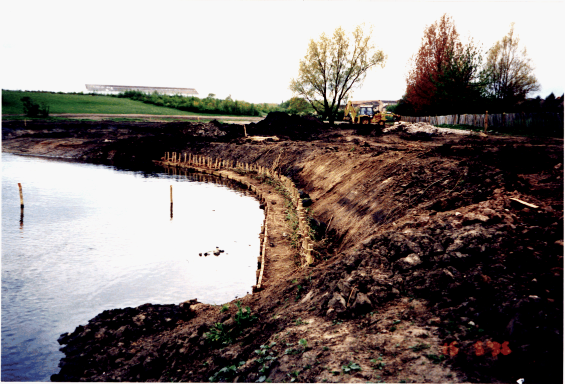
1. Entry spiling - spiling still to complete
