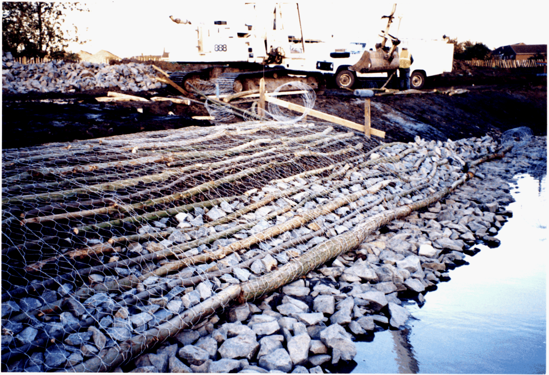
19. Willow mattress in progress
