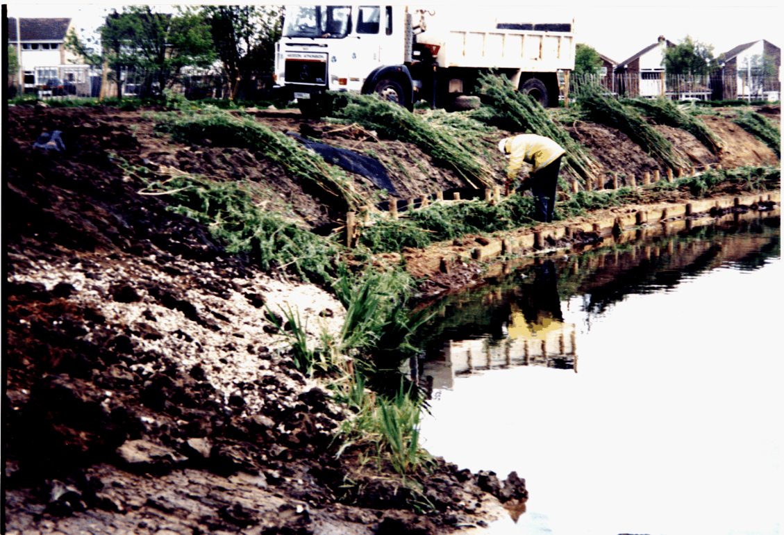
2. Entry spiling - weaving of osier
