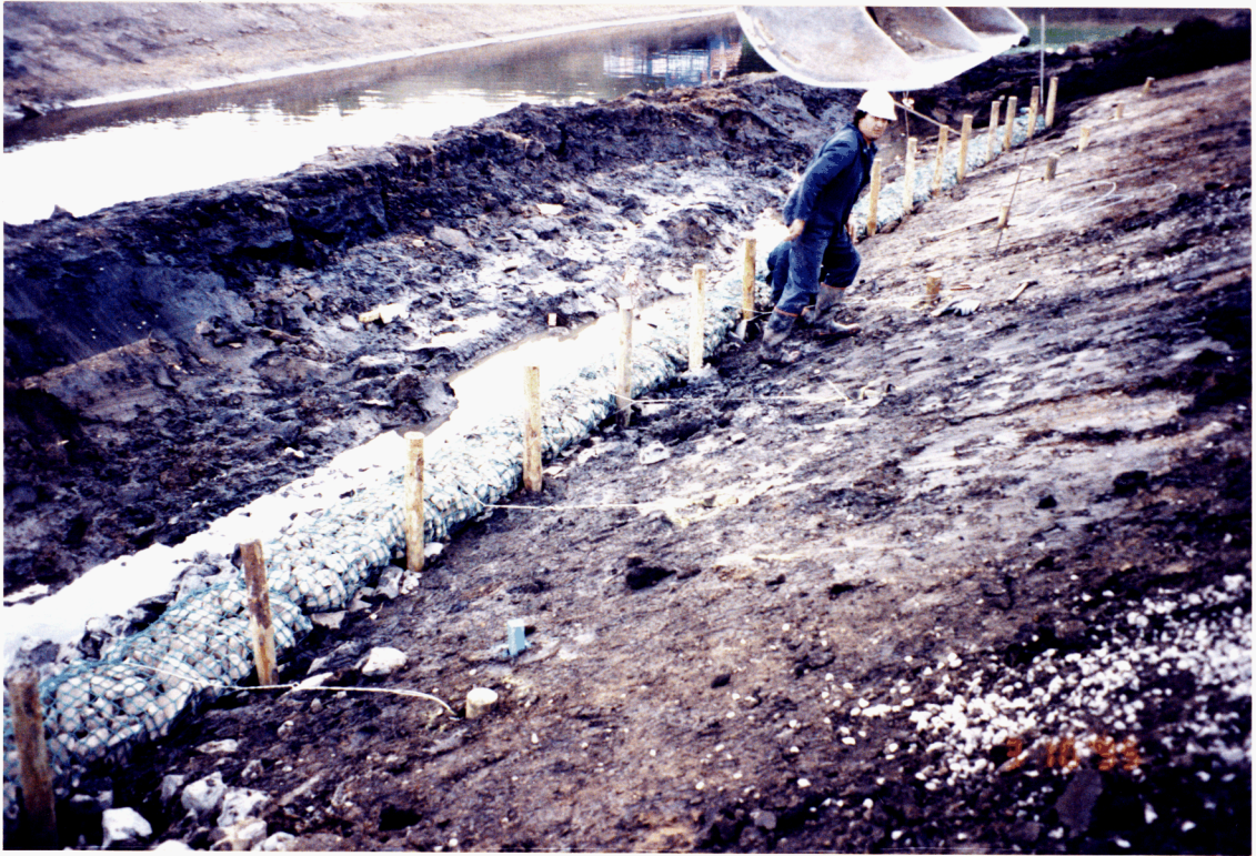
23. Transition rock rolls wired to posts
