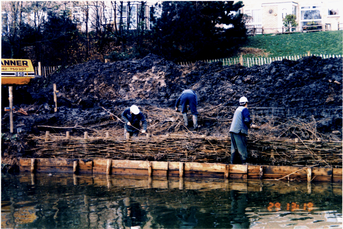
7. Exit spiling - weaving of spiling almost complete
