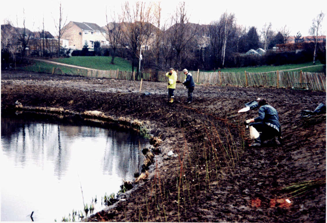
13. Log and geotextile (N3) with willow slips in position
