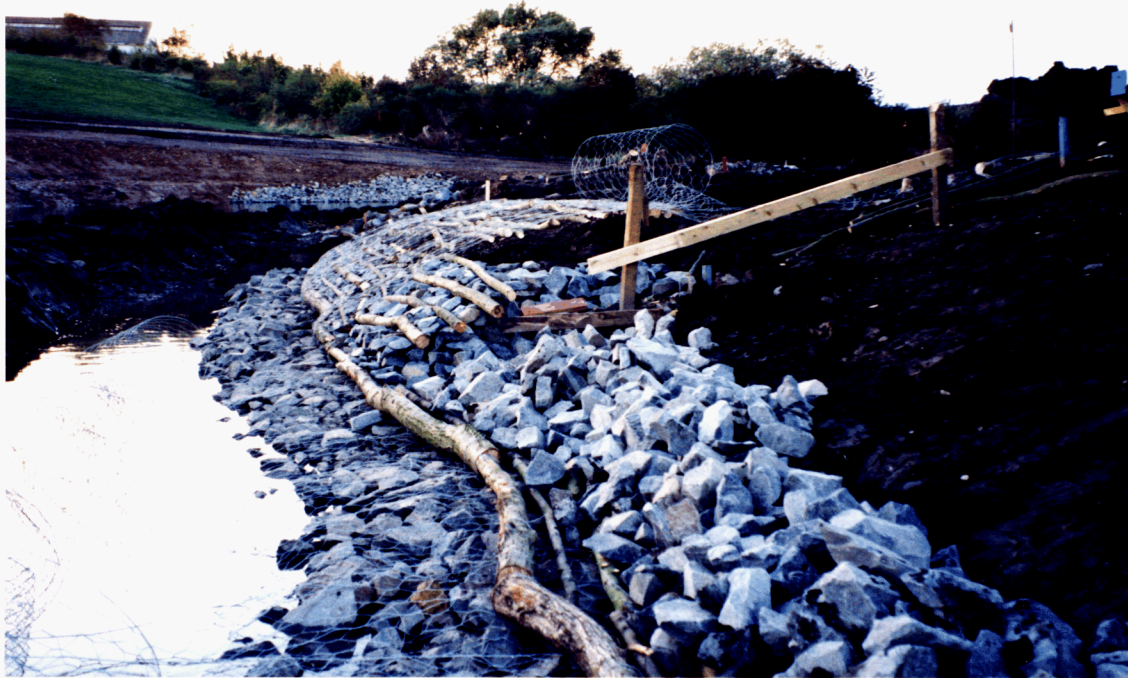
18. Willow mattress - one section under construction
