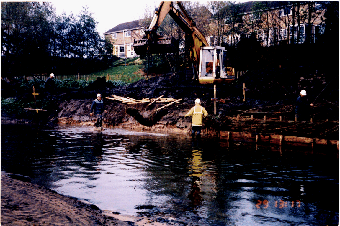
6. Exit spiling - positioning of plant roll
