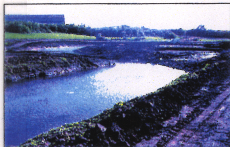
Meanders being constructed
