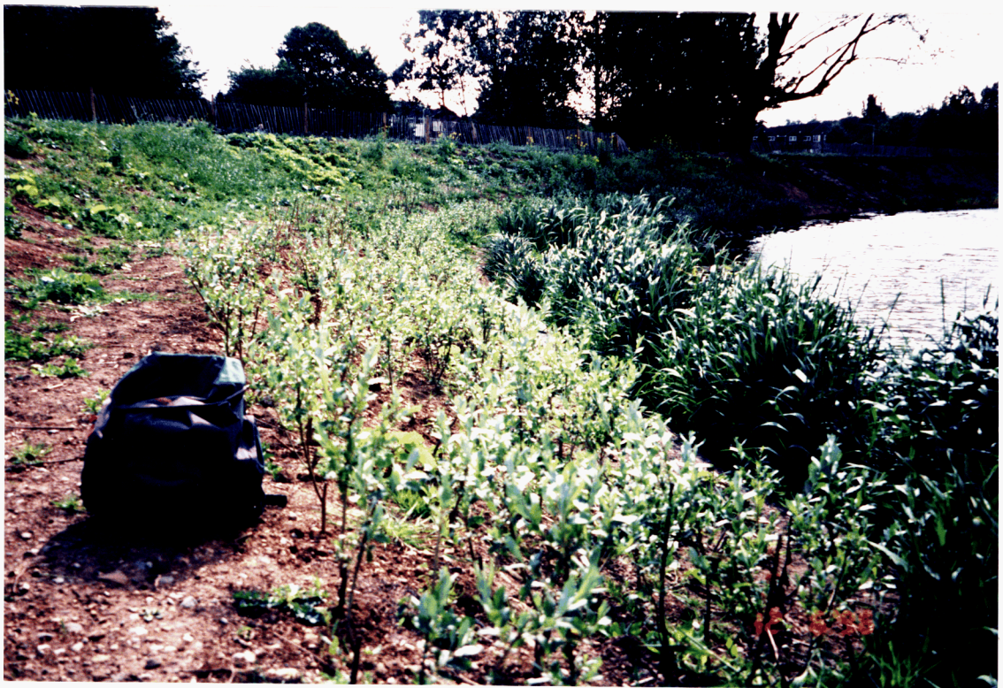
14. Log and geotextile (N1) four months after willows planted
