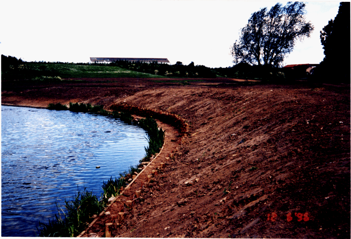
3. Entry spiling complete
