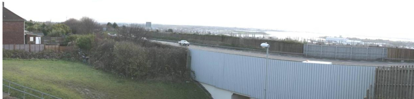
Figure D.11 – POPE OYA view looking south from Hillsley Road: View illustrates former lighting columns now removed and westbound climbing lane.
