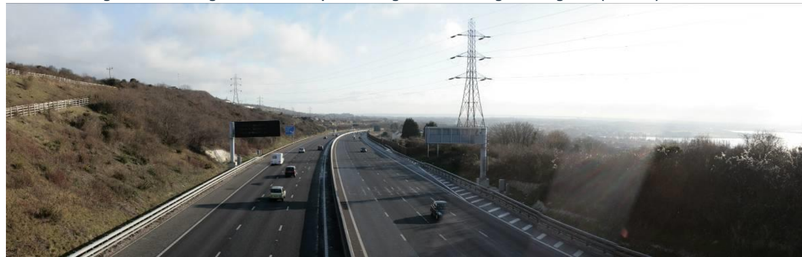
Figure D.8 – POPE OYA view looking east from High Tor footbridge: View illustrates westbound climbing lane, retained signage (eastbound carriageway) and new VMS
