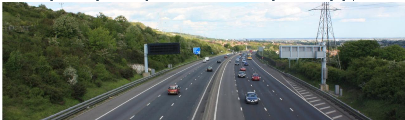
Figure D.9 – POPE FYA view looking east from High Tor footbridge: View illustrates westbound climbing lane, retained signage (eastbound carriageway) and new VMS
