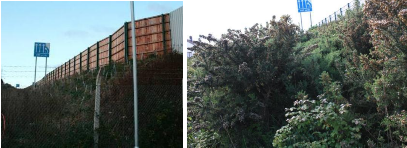
Figure D.13 – Acoustic barrier to the north of Browning Avenue
