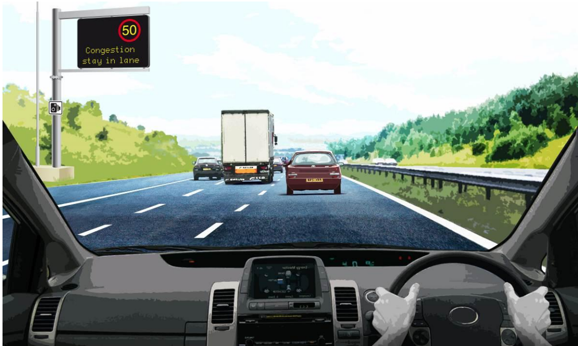
Figure 4D: Illustrative M4 J3 to J12 smart motorway scheme section operating with variable mandatory speed limits and information for road users.
