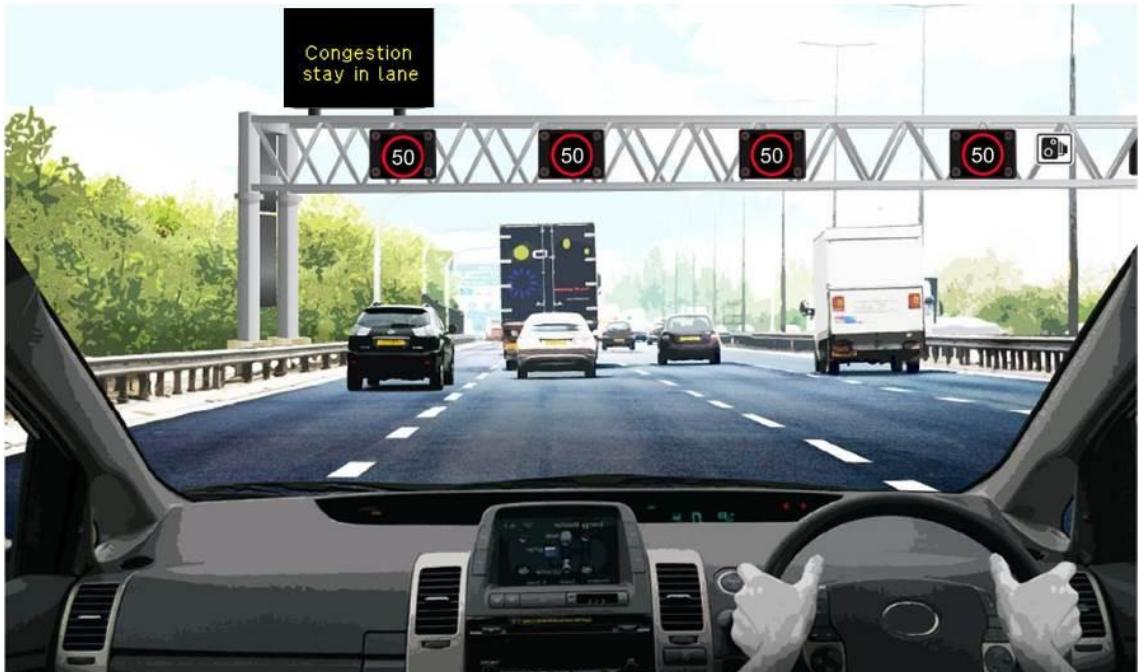
Figure 4C: Illustrative M4 J3 to J12 smart motorway scheme section operating with variable mandatory speed limits
