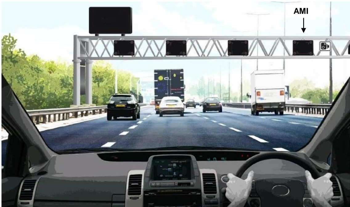
Figure 4A: Illustrative M4 J3 to J12 smart motorway scheme section operating in normal motorway conditions with blank AMI and blank gantry mounted VMS
