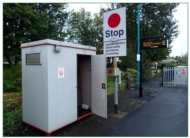
Figure 6: The level crossing control panel partially obscured by the open token hut door
