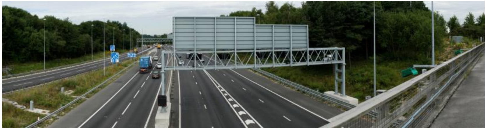
Figure C.10 – POPE OYA View: Changes in gantries are the largest change in the view however relocation of lighting columns from the central reservation can also be seen
