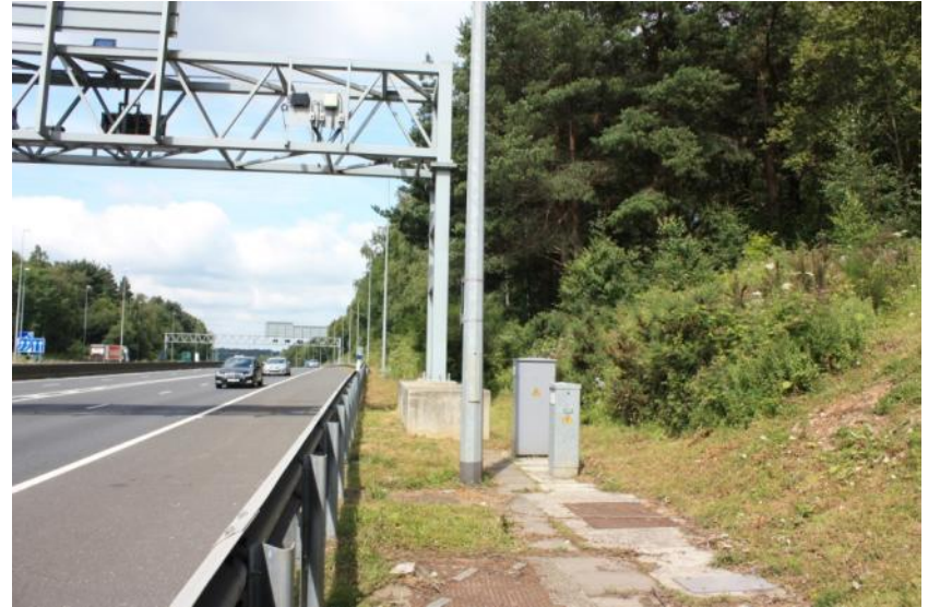
FYA view from access route to service
