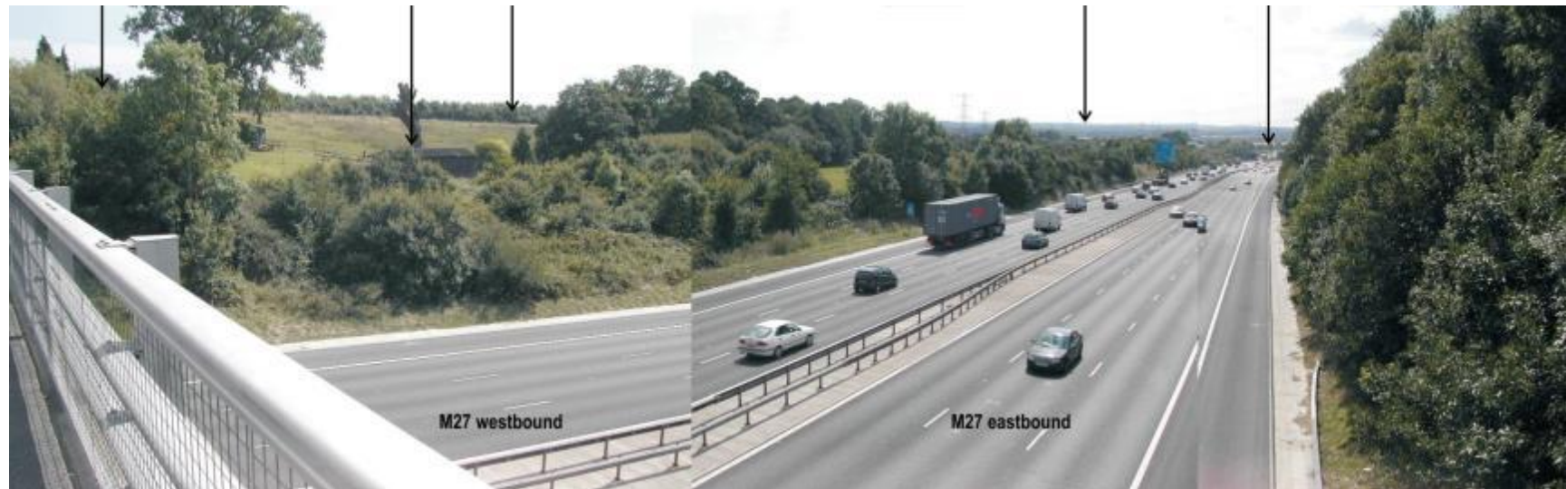
Figure C.28 – POPE OYA View: View illustrates new retaining structure but also how clearance of vegetation to facilitate the widening was kept to a minimum
