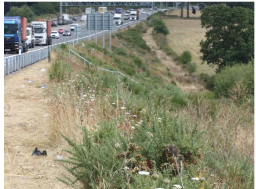
FYA view from motorway looking north east along embankment
