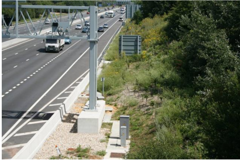
OYA view from bridge
