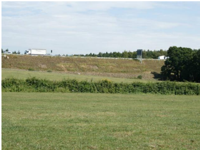
OYA view from footpath towards embankment
