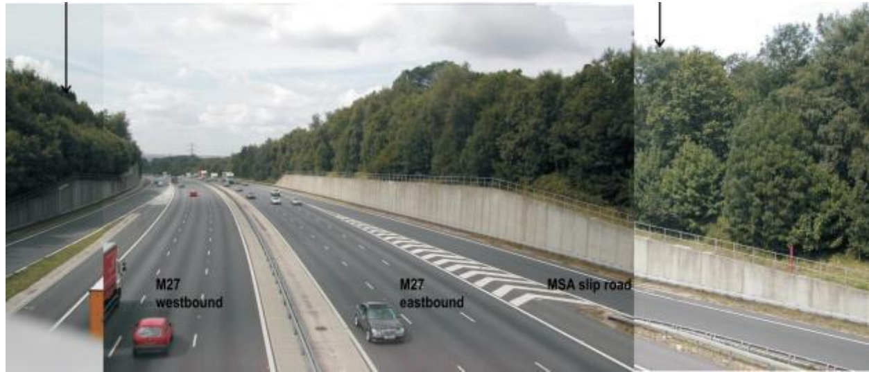
Figure C.7 – POPE OYA view looking south west from the Rownhams Lane overbridge: View illustrates changes to central reservation and introduction of MS4 VMS on the eastbound carriageways
