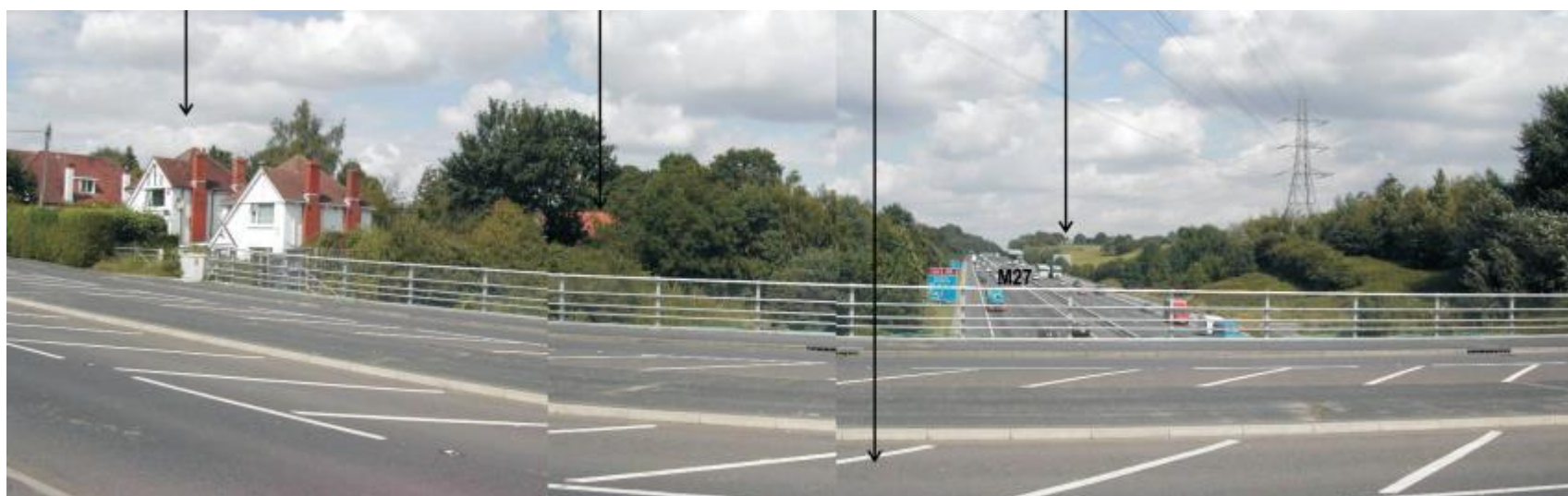
Figure C.25 – POPE OYA View: The new gantry structure is now dominant in the view however retaining structures, loss of vegetation and mitigation planting can all be seen
