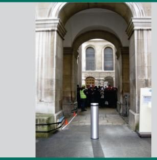
Figure 10: Bollard placed within exit opening (0m stand-off)
