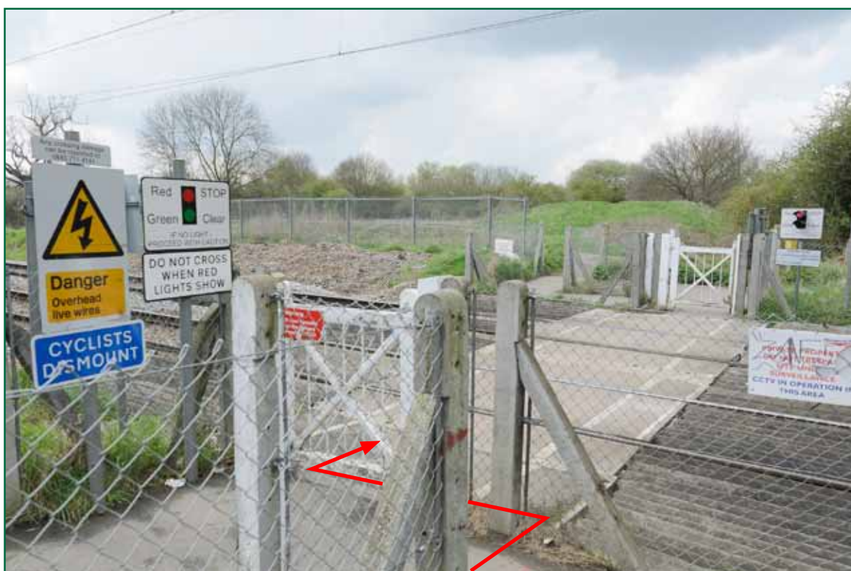
Figure 4: Approach to Johnson's footpath crossing viewed from the east (up) side
