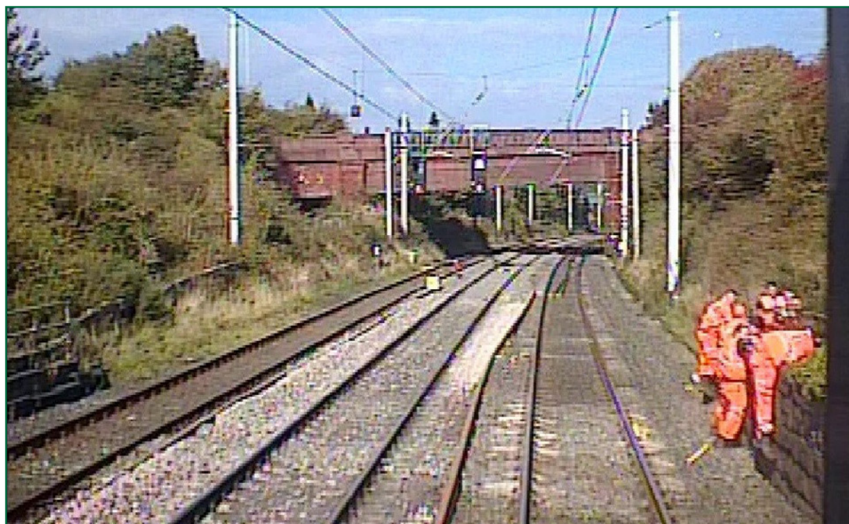
Figure 10: Image of workgroup from rear-facing CCTV camera fitted to train 1M97 showing yellow jack beneath right-hand rail (courtesy of FTPE)
