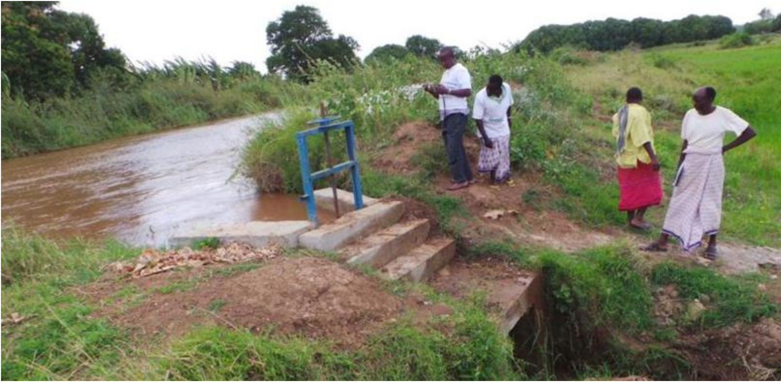
Sluice gate in Halgan village. Photo taken on September 5 th 2014.
