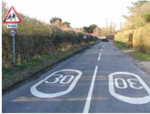
Figure 22: These speed limit roundel repeater road markings are unnecessary in a rural conservation area. Their shape is also unlawful (they must be circular) so they must be removed
