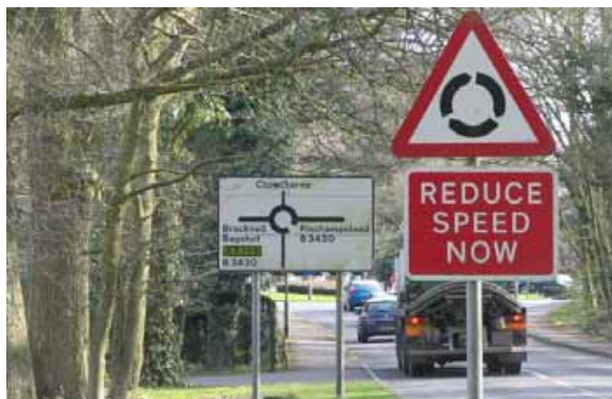
Figure 13: This warning sign obscures long distance visibility of the larger directional sign from oncoming drivers
