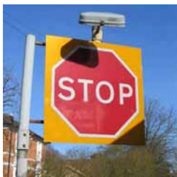
Figure 30: Obtrusive yellow backing board in an urban conservation area
