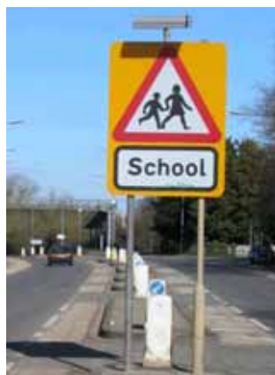
Figure 24: Large school warning sign with yellow backing board on a 40mph road – too large for its environment or justified because of the risk?
