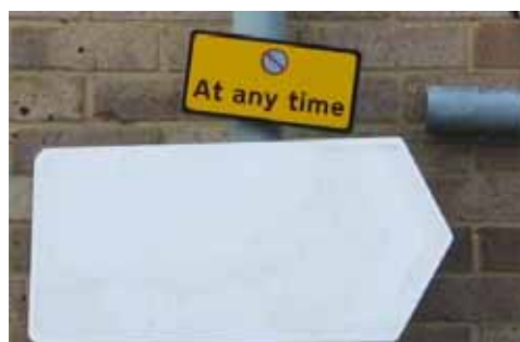
Figure 20: These signs are either obsolete or unreadable and must be removed
