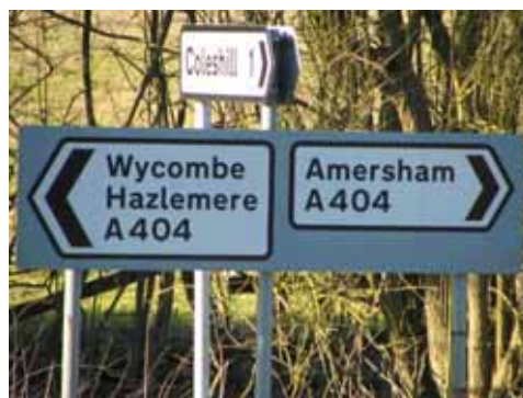
Figure 33: Appropriate use of grey backing board for mounting flag type direction signs
