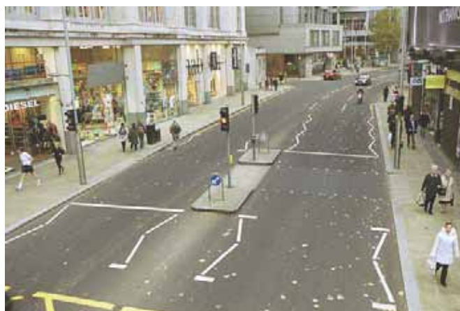
Figure 1: Kensington High Street – minimal zig-zag markings (Awaiting permission for use from RB Kensington and Chelsea)
