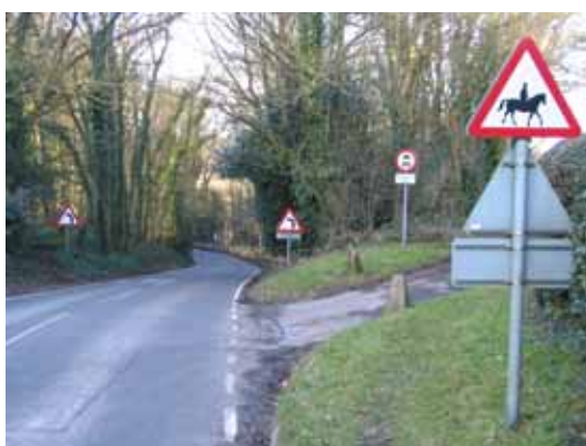
Figure 14: Excessive number of warning signs on a rural lane
