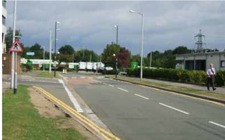
Figure 16: There is an unobstructed long distance view of this zebra crossing, but the sign is set too far away from the road where it may not be seen
