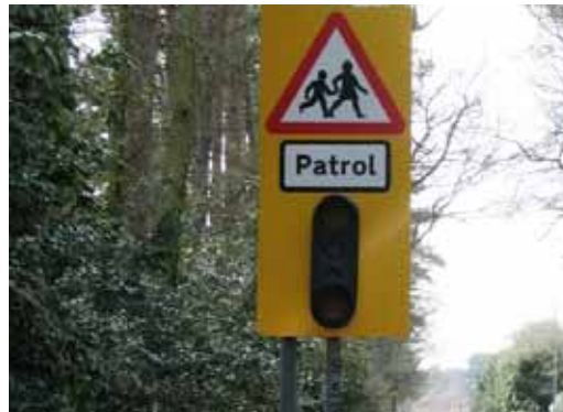
Figure 32: This yellow backing board is unnecessary and it reduces the contrast between the yellow flashing light and the background
