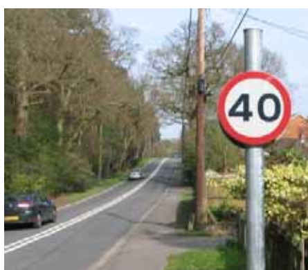
Figure 28: Sign post protruding above the top of the sign
