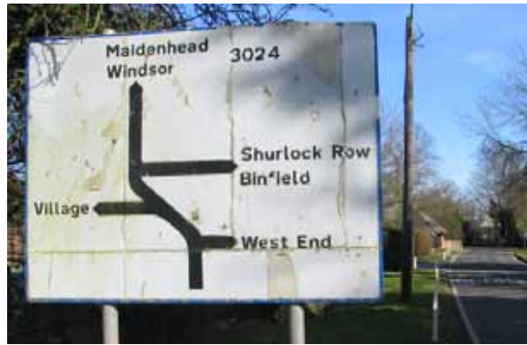
Figure 25: Apart from its poor condition, this sign is oversized for its rural environment. The layout is also unsuccessful as it does not make efficient use of the sign space.
