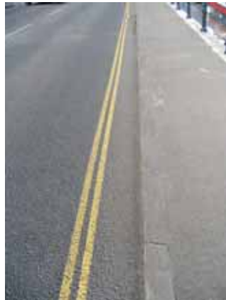
Figure 36: Use of narrow double yellow lines in a conservation area
