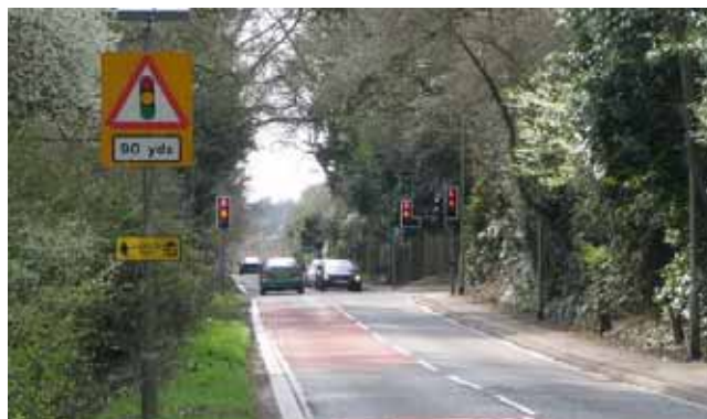
Figure 15: Traffic signal warning sign positioned close to signals – with a higher level of illumination, the signals can be seen from further away than the sign by day and night
