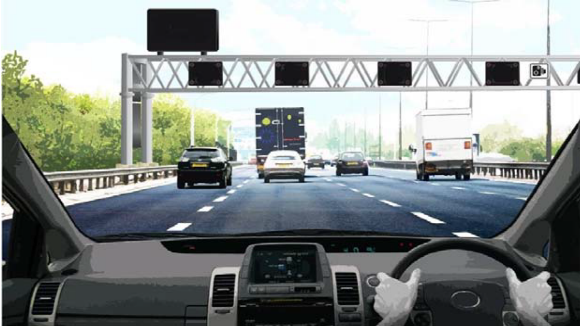
Figure 3C: Illustrative MM-ALR section operating in normal motorway conditions with blank Advanced Motorway Indicators and blank gantry mounted Variable Message Sign
