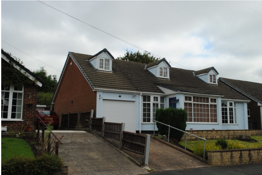
Source: BRE photo library
