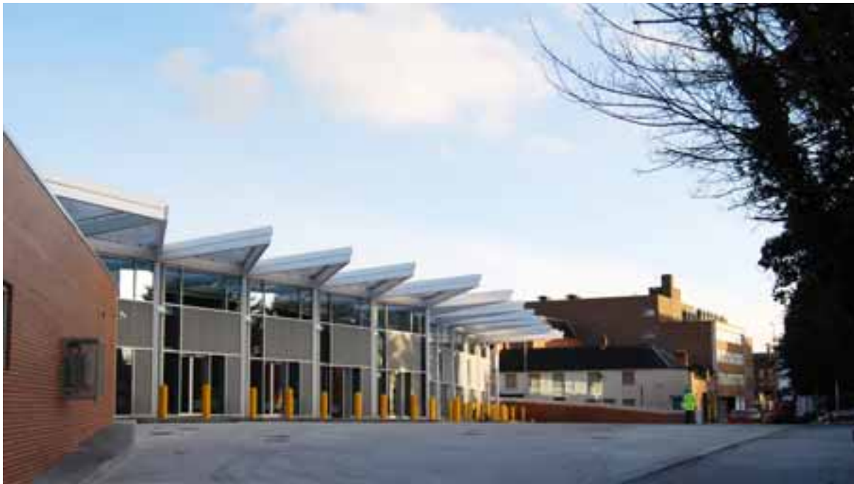
North Gate Bus Station, close to completion
