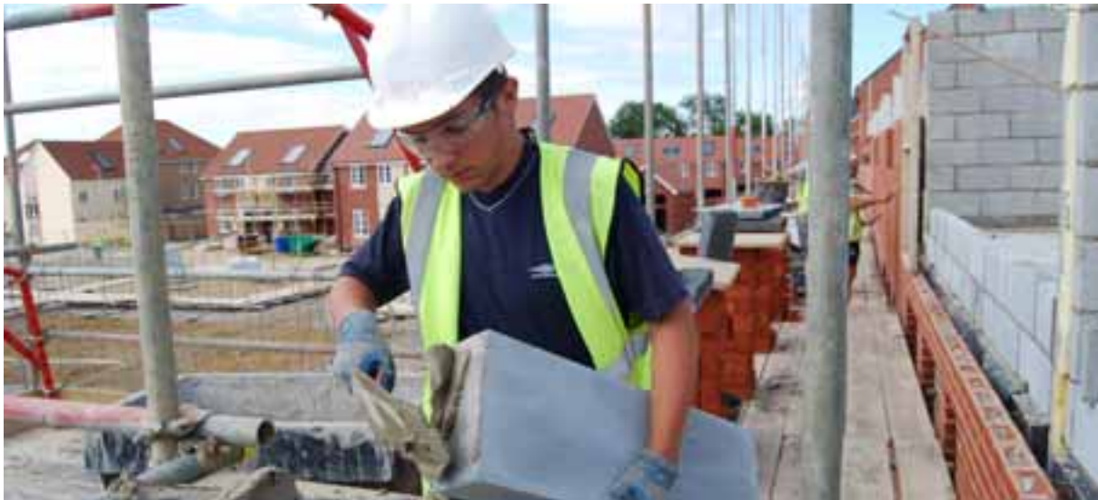
David Tompkins, Construction Futures trainee
