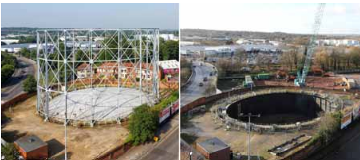
St Peter's Way Gasholder before and after demolition
