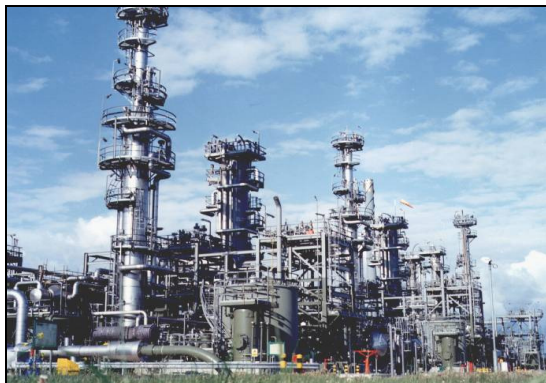
Photo 5 - POA Gas Terminal
