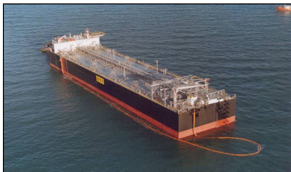
Photo 4 - Oil Storage Installation
