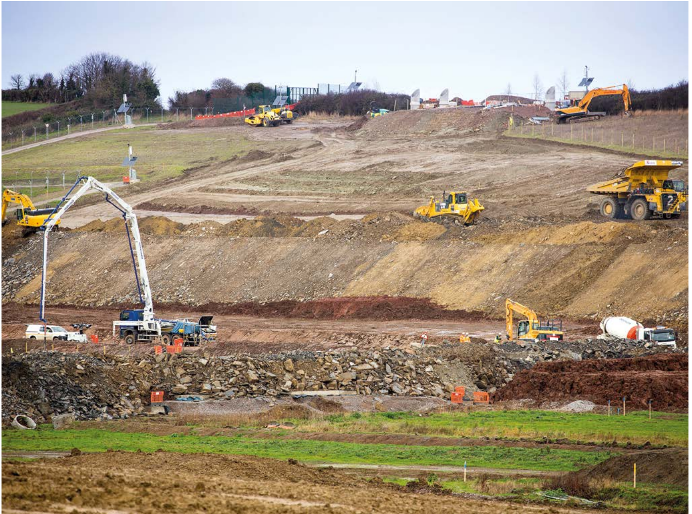
Above: site preparation work at Hinkley Point C
