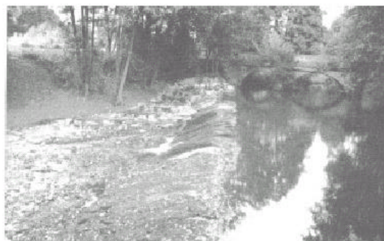
Figure B.22: Plan view of a fish ramp in the corner of a weir on the Elz River, Germany (after Gebler, 1998)
