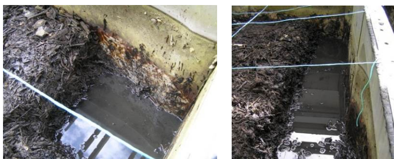
Figure 36. Excavation of the upper layer of compost substrate
