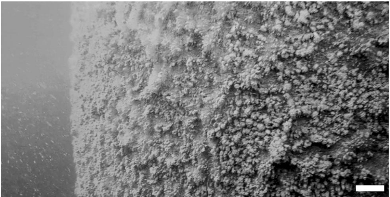
Fig. 5.22: Monopile fouling at the Belwind I OWF 7 months after piling.
