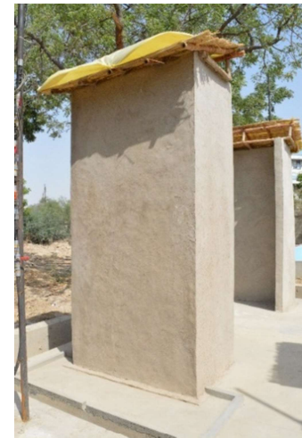
Figure 6. Wall to be tested
