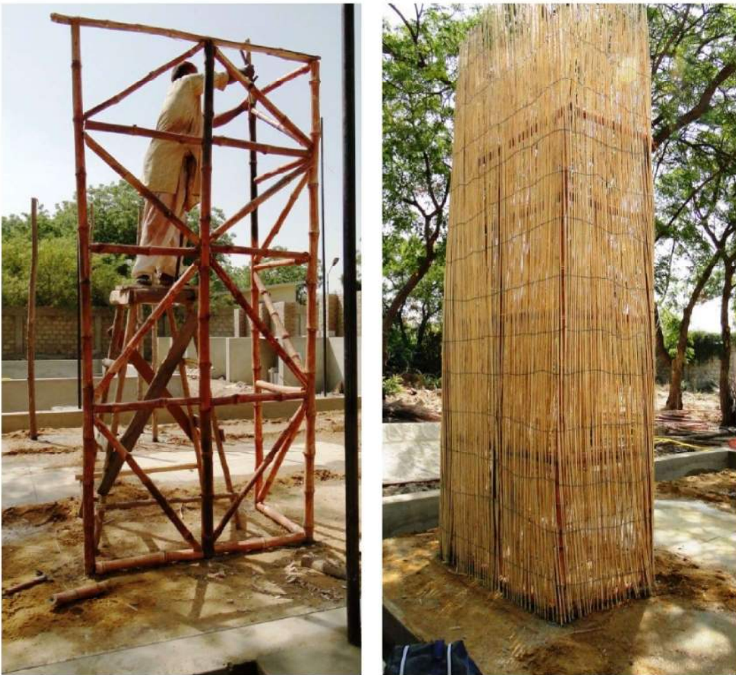
Figure 4 Loh-kat panel at testing facility made from bamboo frame and chicks matting. The next step is to apply plaster to the chicks matting. Note that the bamboo frame requires lots of diagonal bracing in order to make it stable. With many loh-kat shelters recorded as visibly leaning over it is most likely due to insufficient bracing.
