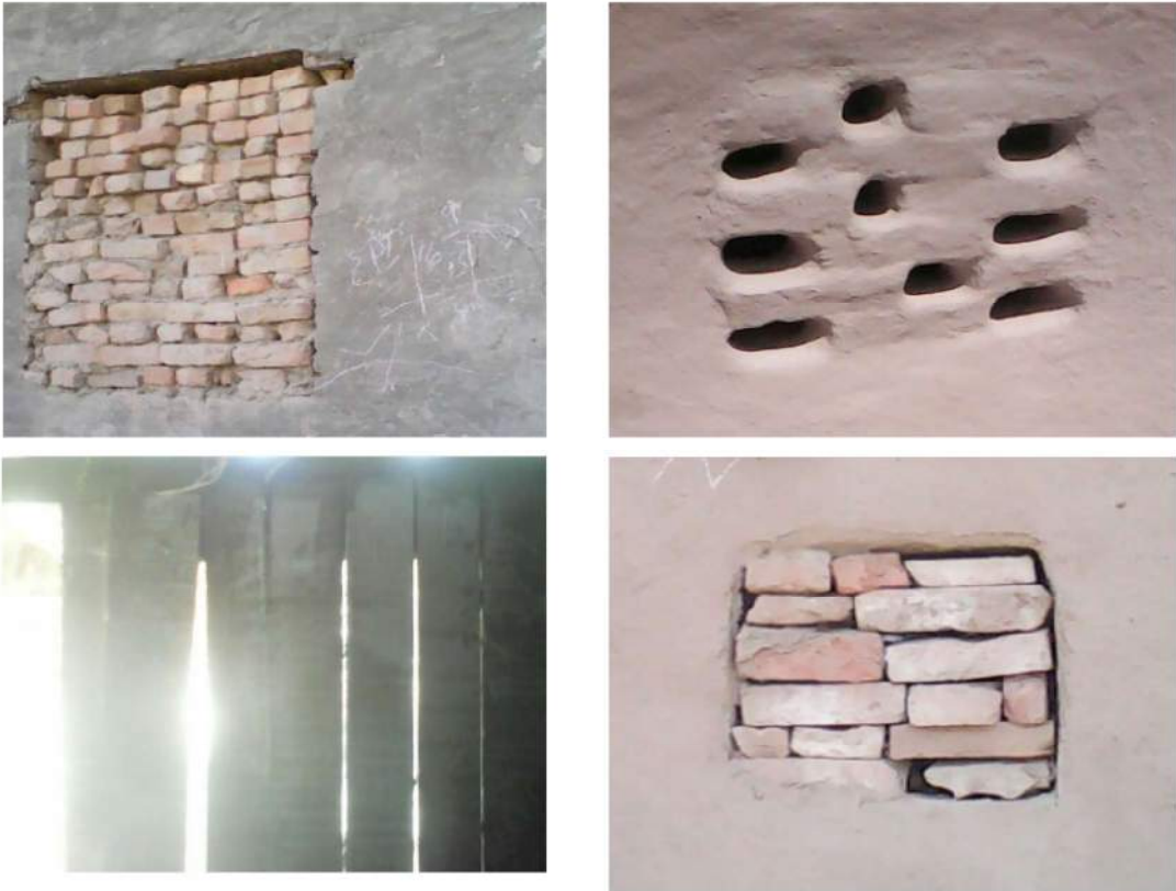
Figure 19 - Modifications made to windows by homeowners seeking to address concerns over privacy and
