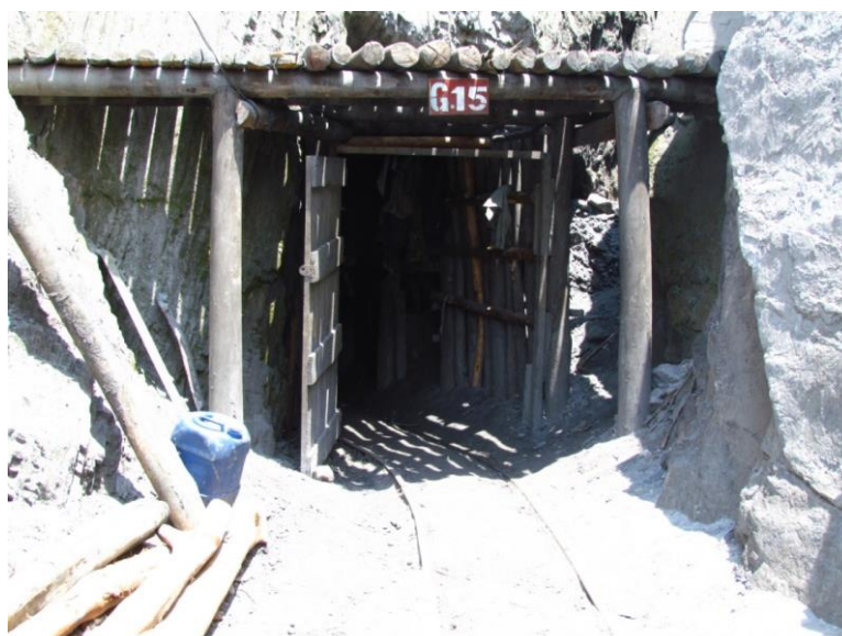
Figure 34: Tunnel G15 in Gifurwe
