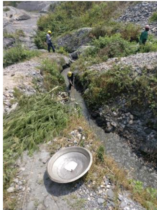
Figure 39: WMP river sluicing
