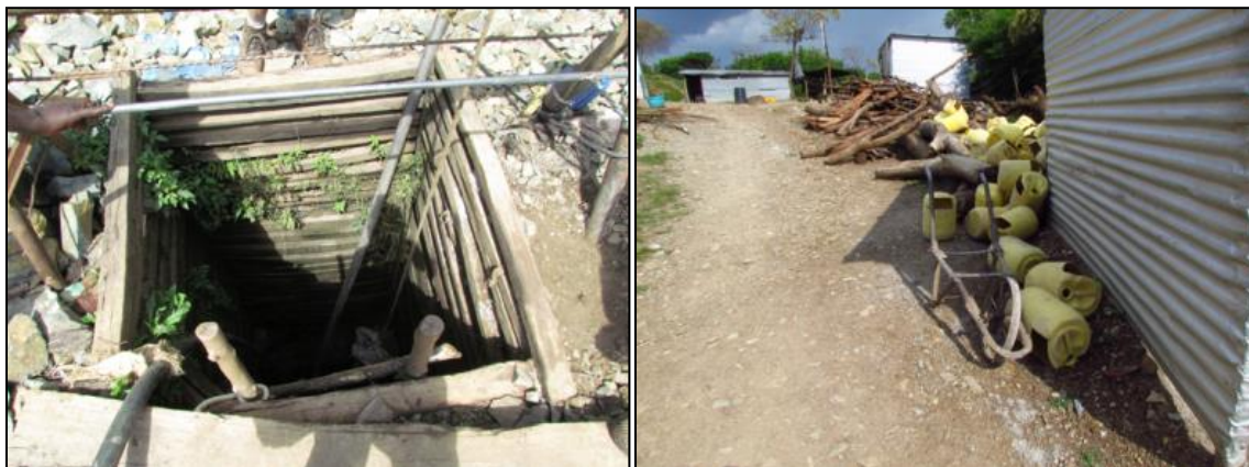
Figure A37: (left) Although well-timbered, this shaft is plagued by frequent flooding; (right) Wood used for underground timbering is stacked next to discarded drums used to haul ore from depth
