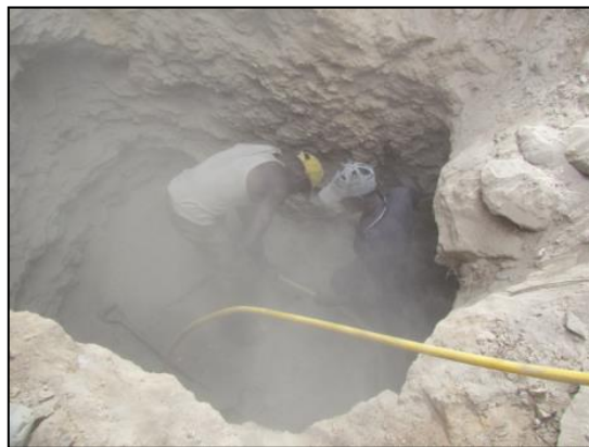
Figure 22: Dust exposure during dry rock breaking with jackhammers
