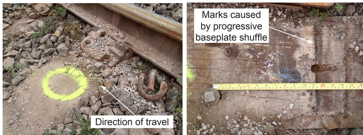
Figure 8: Views before and after removal of right-hand baseplate at bearer no. 0
