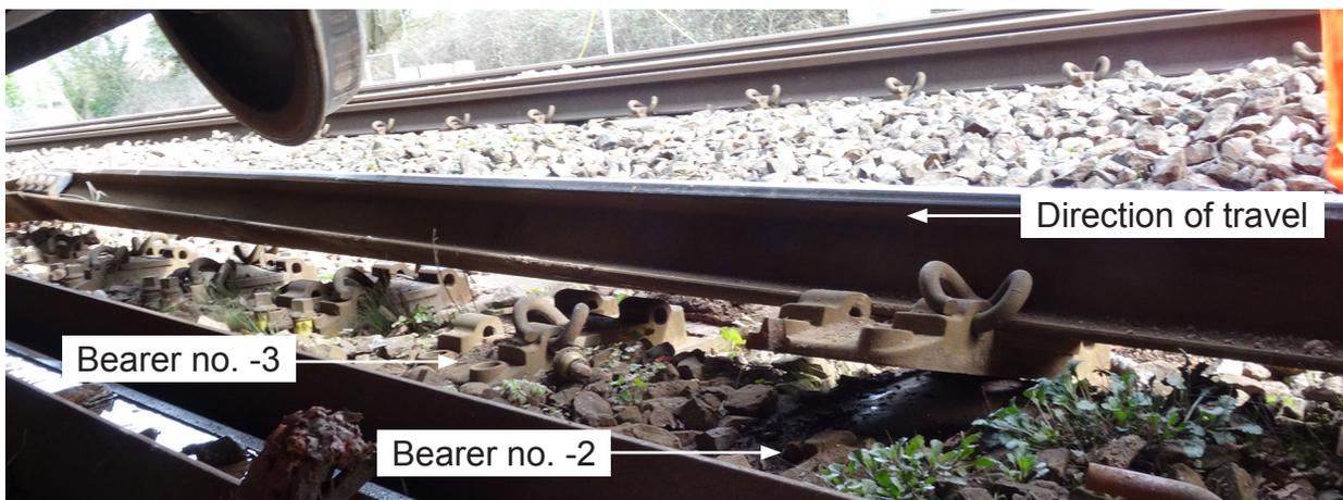
Figure 10: View showing outwards rotation of the right-hand rail
