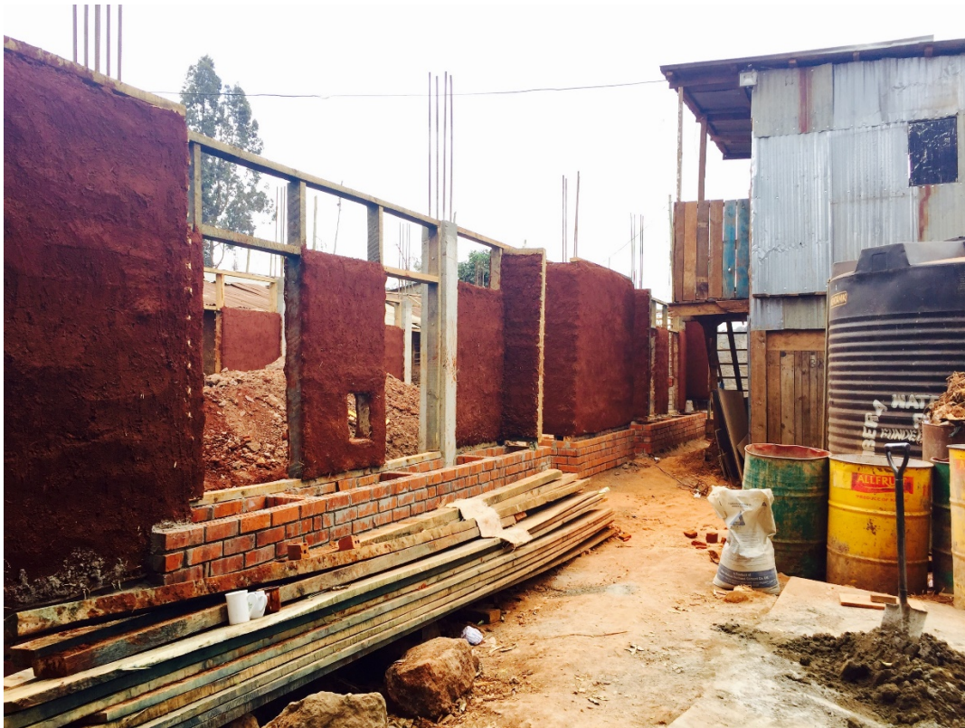
Photo 3: Mud construction at KDI's ANWA school upgrading project site, Kibera, 2016.
