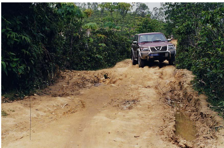
Figure C.1 - Rural gravel road in Vietnam lacking maintenance.
