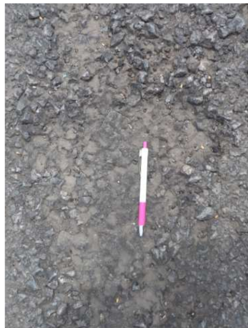
Figure A.21: Centre-line pothole and close up of new pothole forming on right (exposed primed base)
