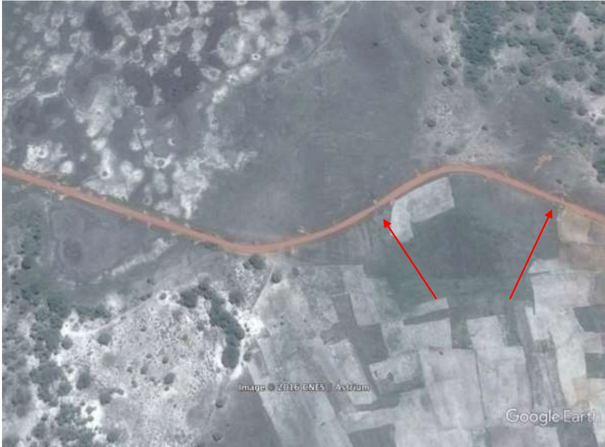
Figure B.30: Road R451 crossing between two marshy areas with only two culverts. The closely spaced mitre drains on the left have been installed after 2013
