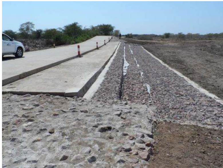
Figure B.14: Concrete drift with stepped gabion basket
