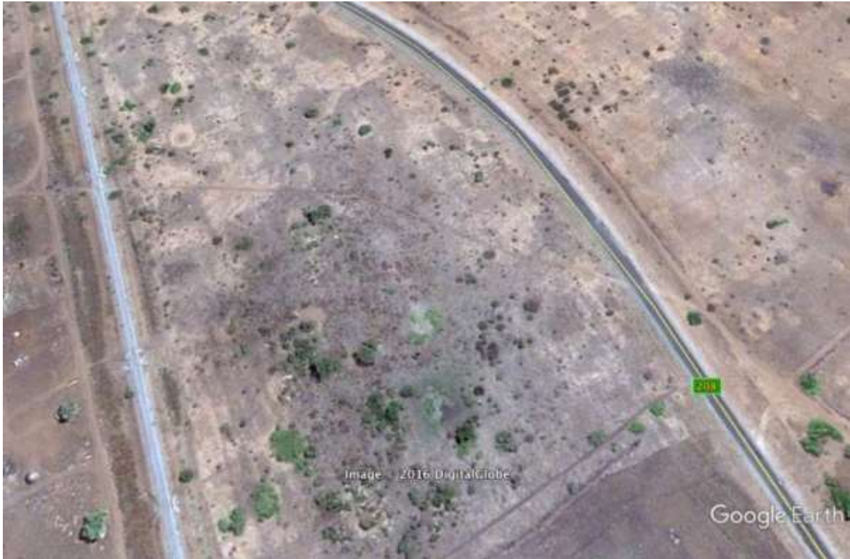
Figure 27: Google Earth image of road and railway line comparing cross-drainage structures
