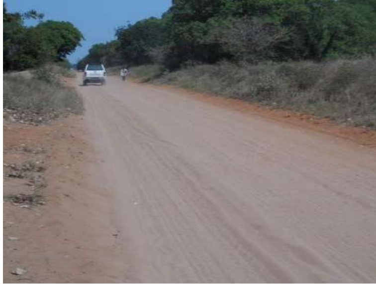
Figure B.28: Typical example of road prior to upgrading
