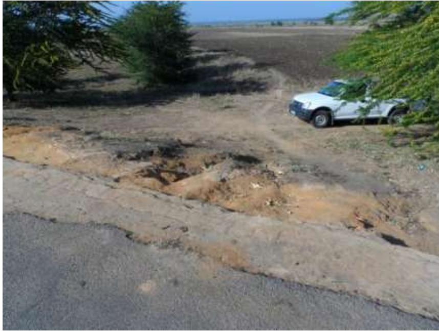
Figure B.6: Erosion of track caused by vehicle movements
