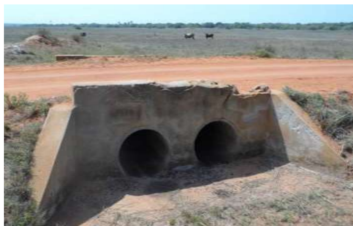
Figure B.31: Typical example of road prior to upgrading
