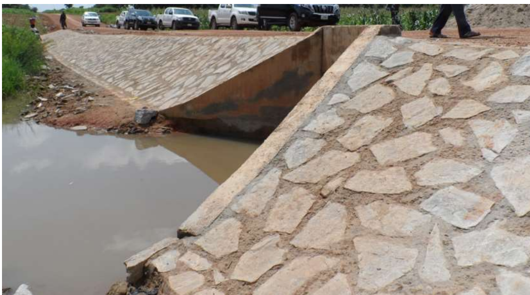
Figure 40: Stone pitching to avoid erosion around culvert wing-walls
