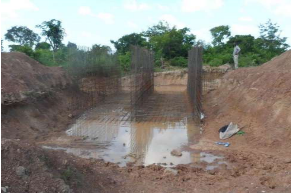
Figure C.3: Construction of standard double 2 x 2 m reinforced concrete box culvert
