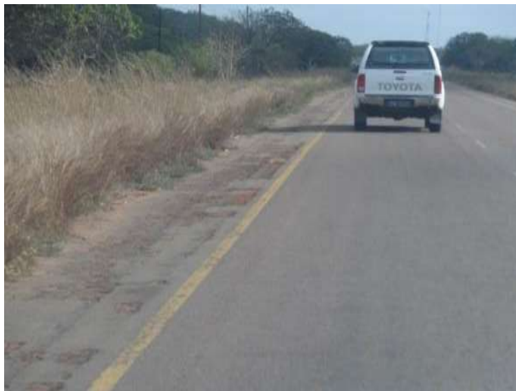
Figure B.33: Example of failure of non-durable single seal on shoulder
