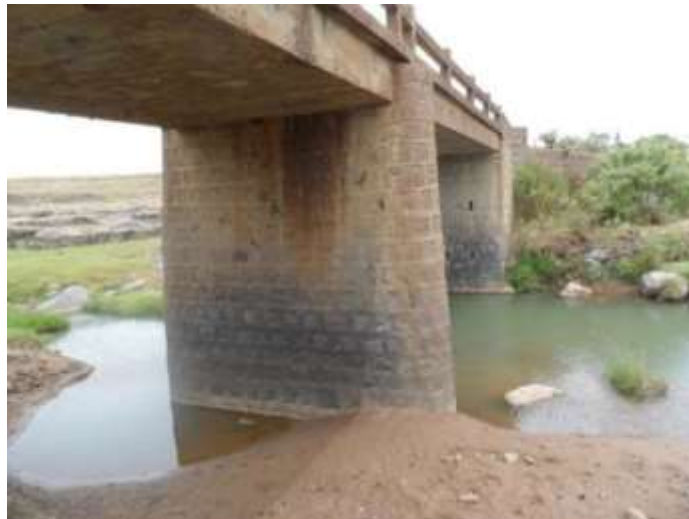
Figure A.7: Bridge at km 8.1
