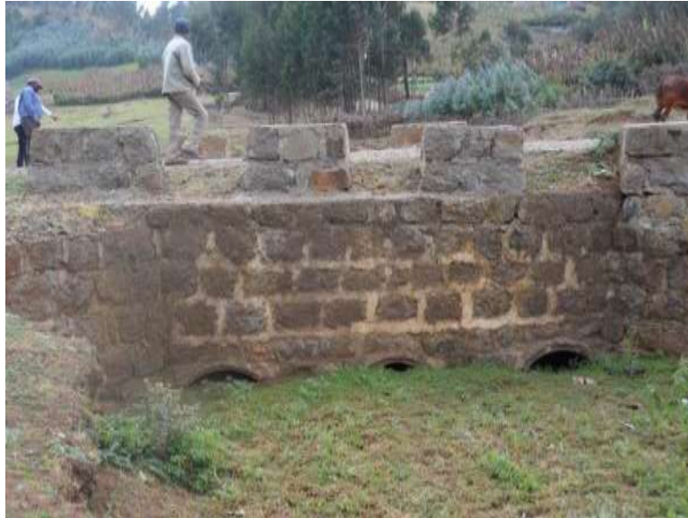
Figure 16: Upstream view of diversion channel
