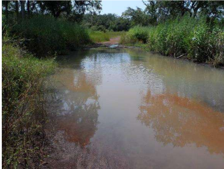
Figure C.20: Newly constructed culvert in flat terrain
