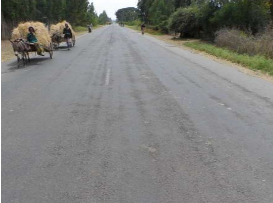
Figure A.20: Streaky nature of the double seal
