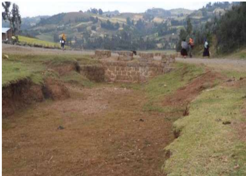
Figure 15: Construction of a river diversion (downstream side view)
