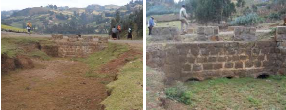
Figure A.14: Diversion channel and culverts
