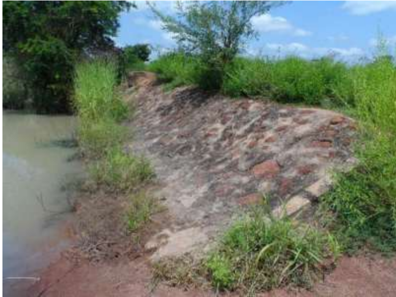
Figure C.10: Grouted stone pitched embankment protection
