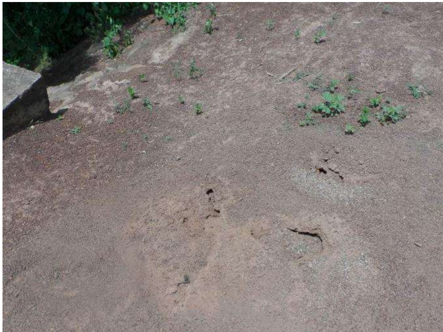
Figure C.11: Initiation of ant nest in embankment
