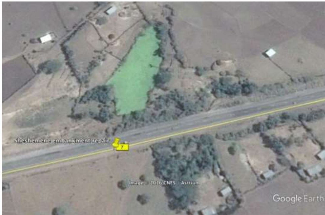
Figure A.24: Google Earth image of problem area near Sheshemene (23/2/2016)
