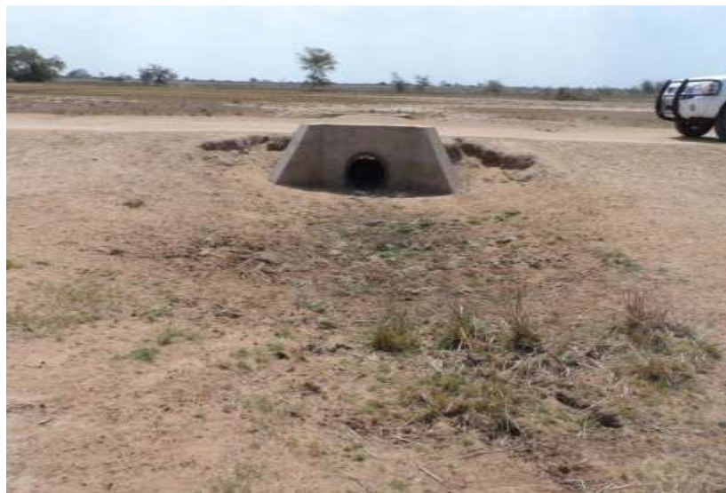
Figure B.16: Newly constructed culvert in flat terrain
