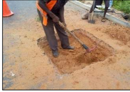
Excavation of Test pit on LTPP 2
