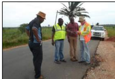
Demonstration of detailed Visual Assessment and collection of data for further analysis
