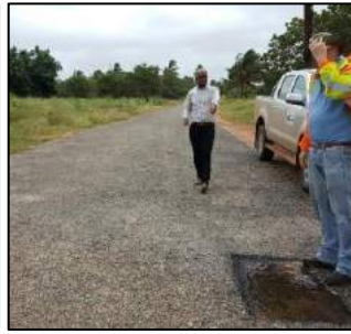
2 nd Experimental Section; Penetration Macadam on Sand Base
