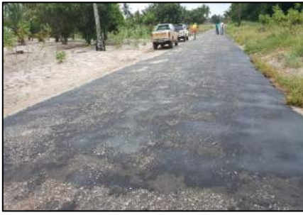
1 st Experimental Section; Sand Seal on Armoured-Calcrete-Sand Base
