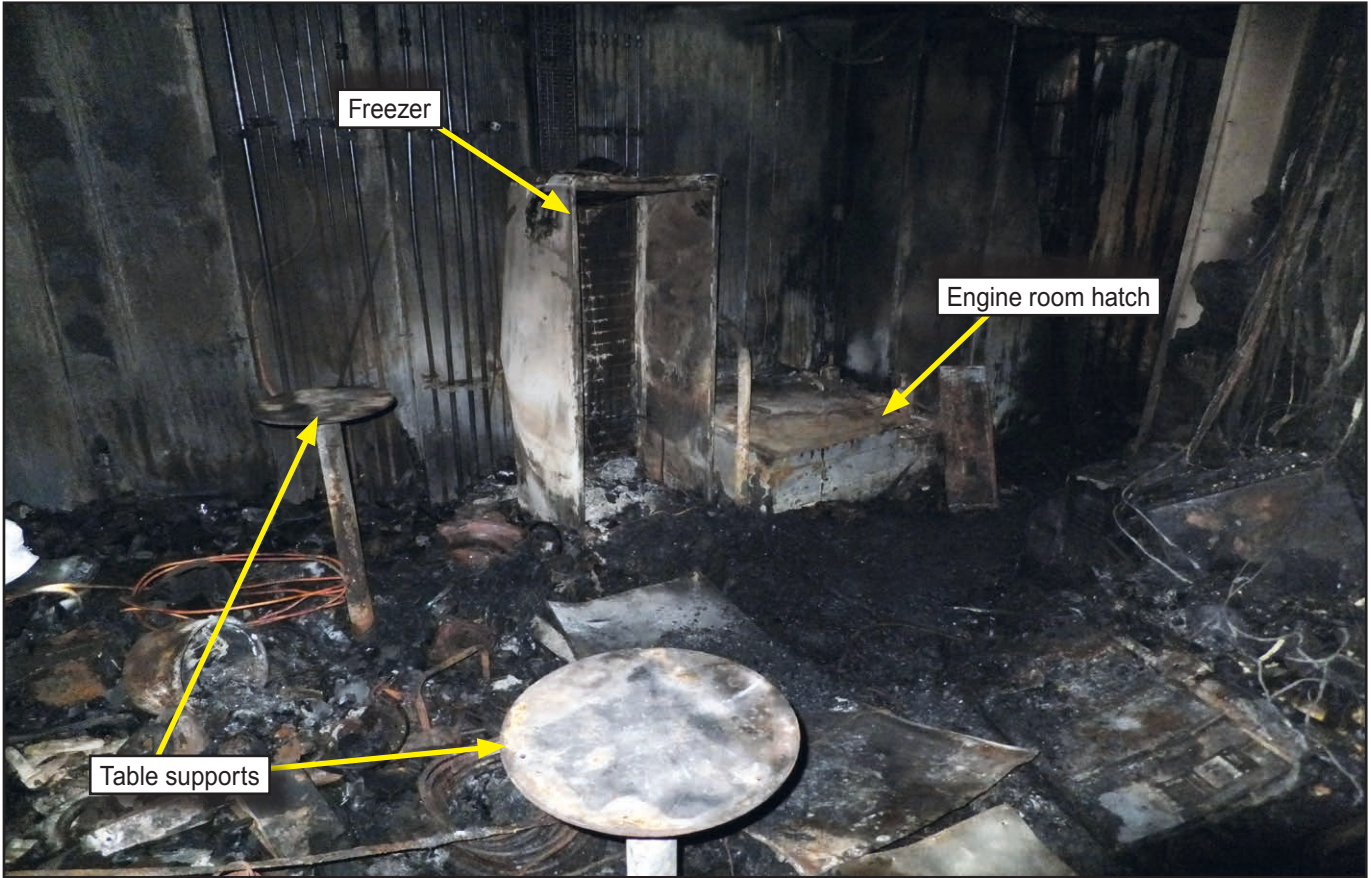
Figure 4: Fire damage to crew mess room
