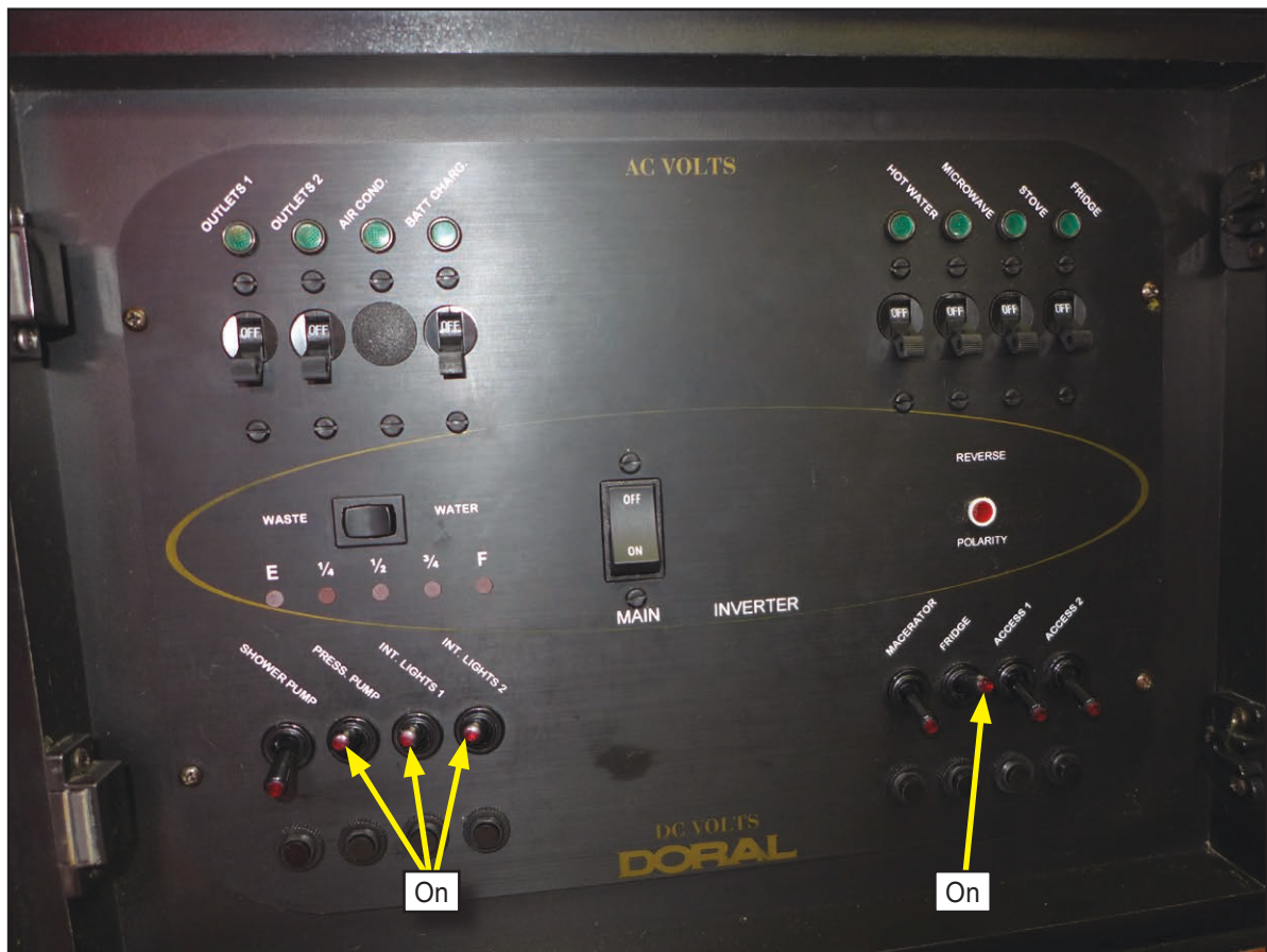
Figure 11: Power distribution panel
