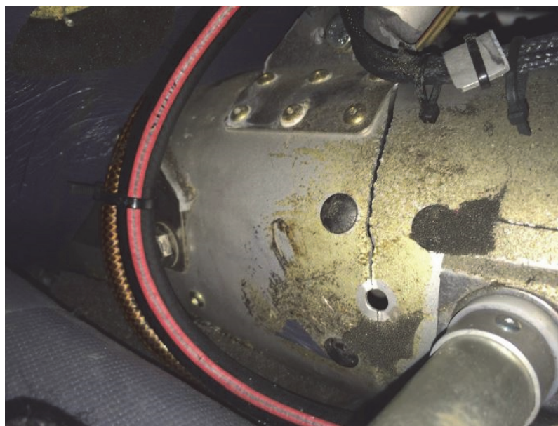
Figure 5b Example of crack emanating from rear cut-out, as shown in OSB 29
