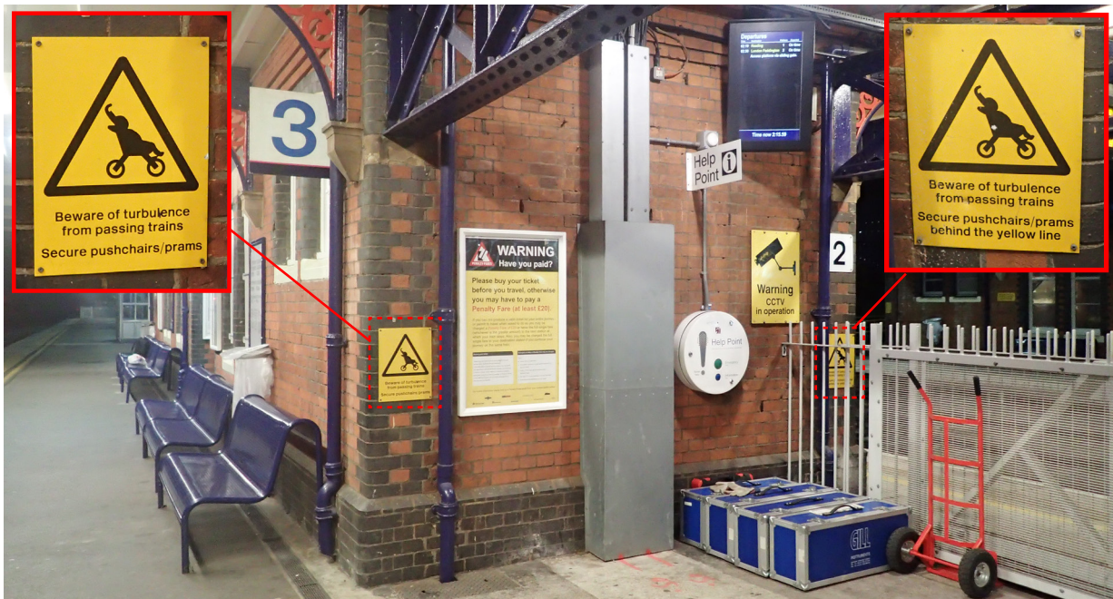
Figure 15: Warning signs on platforms 2 and 3
