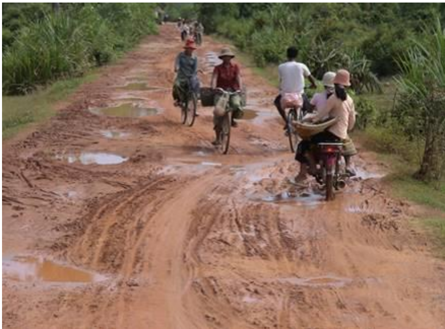
Figure 5.1 - Rural gravel road in Cambodia after one rain season and without maintenance.
