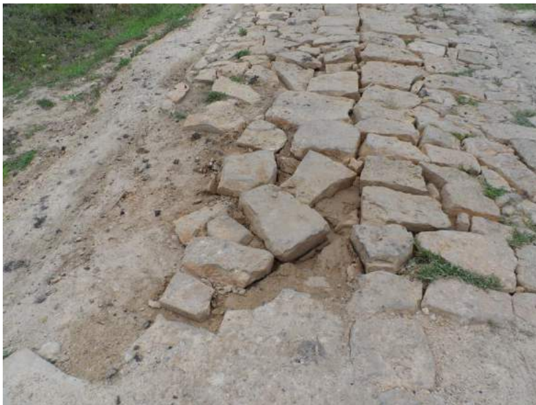
Figure 17: Damage to hand-packed stone road after flooding
