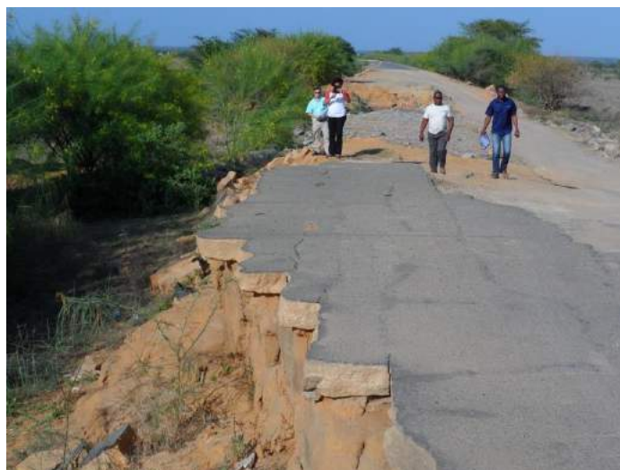
Figure 19: Undercutting and collapse of pavement due to erosion of embankment
