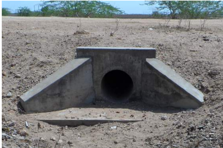
Figure 40: Separation of wing-walls from headwall on relatively new culvert
