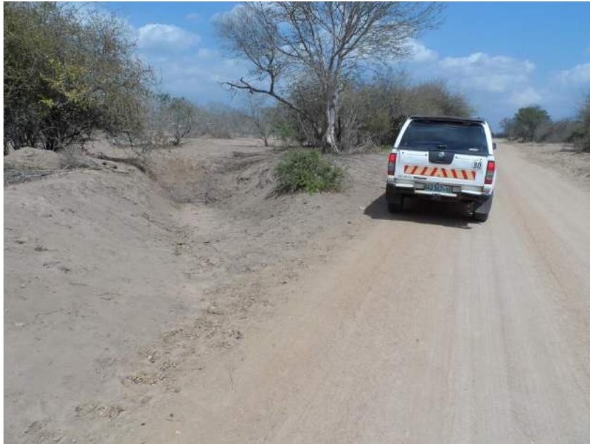
Figure 35: Short mitre drain that is unable to dissipate collected water effectively
