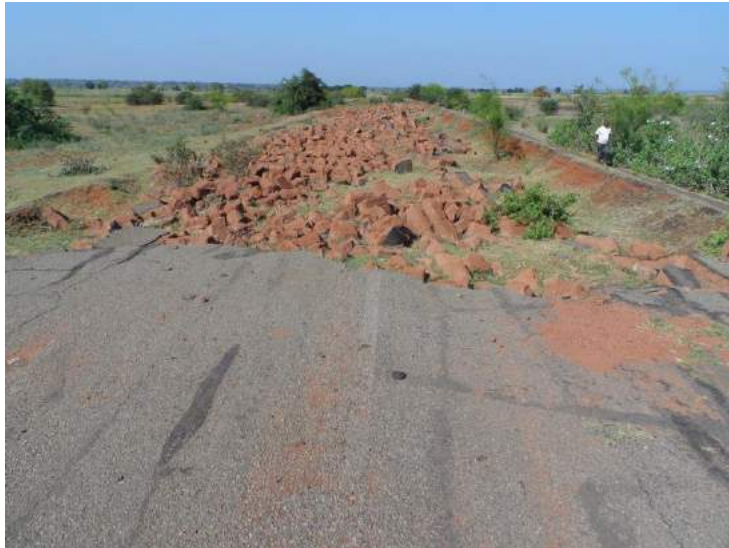
Figure 20: Complete loss of embankment and road due to turbulent flow conditions during overtopping and weak subbase
