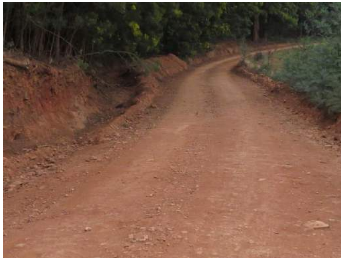
Figure 10: Typical engineered earth road showing shaped structure and side drains
