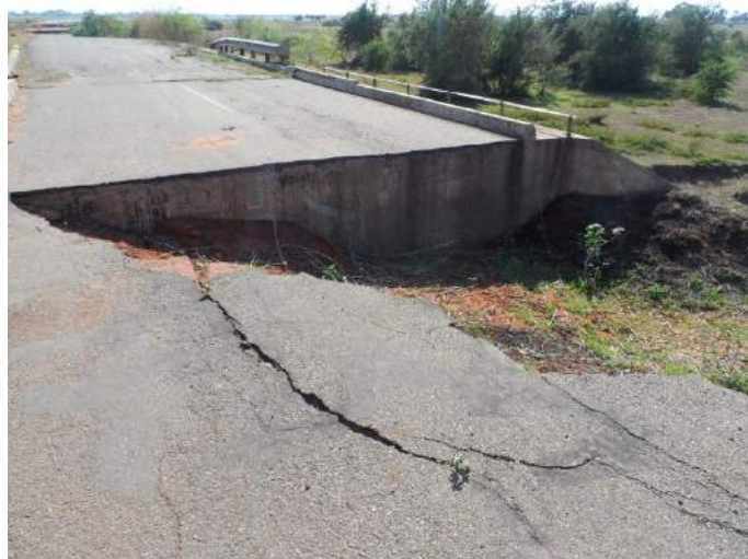
Figure 36: Flood damage to bridge abutment after overtopping of embankment
