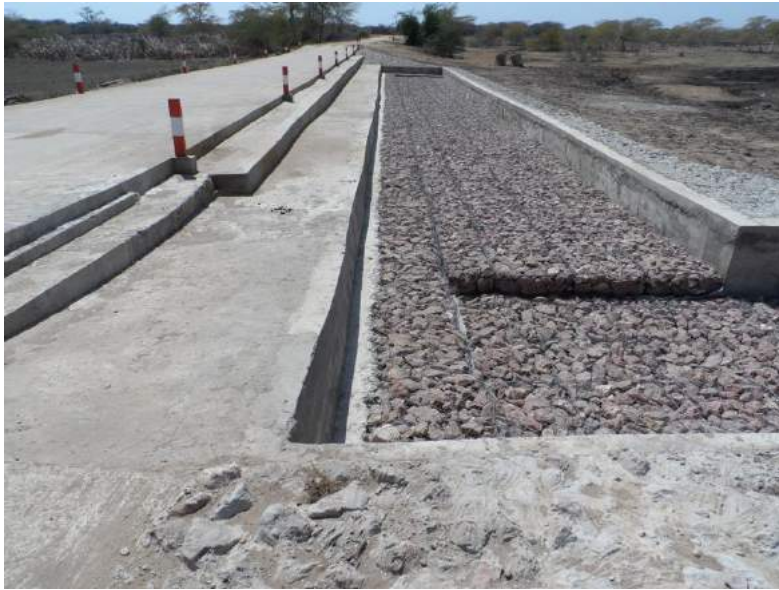
Figure 23: Complex concrete ford with water velocity controllers and stilling pond
