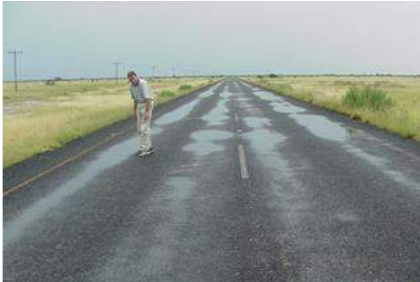
Figure 33: Typical manifestation of collapsible subgrade
