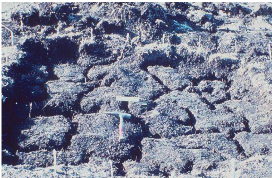
Figure 26: Typical evidence of the presence of expansive clay soils
