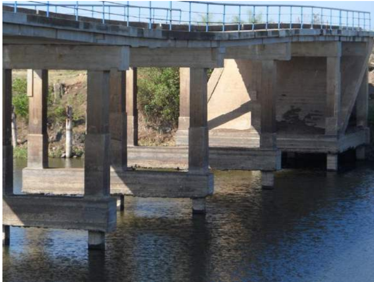
Figure 38: Subsidence of bridge deck due to scour damage of support pier
