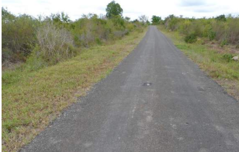
Figure 34: Grassed and built-up shoulders negating effectiveness of drainage from road surface
