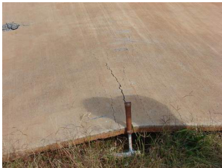
Figure 16: Lifting of thin continuously reinforced concrete road resulting from thermal expansion
