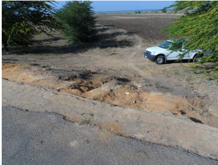
Figure 24: Erosion cause by access of vehicles and pedestrians off road
