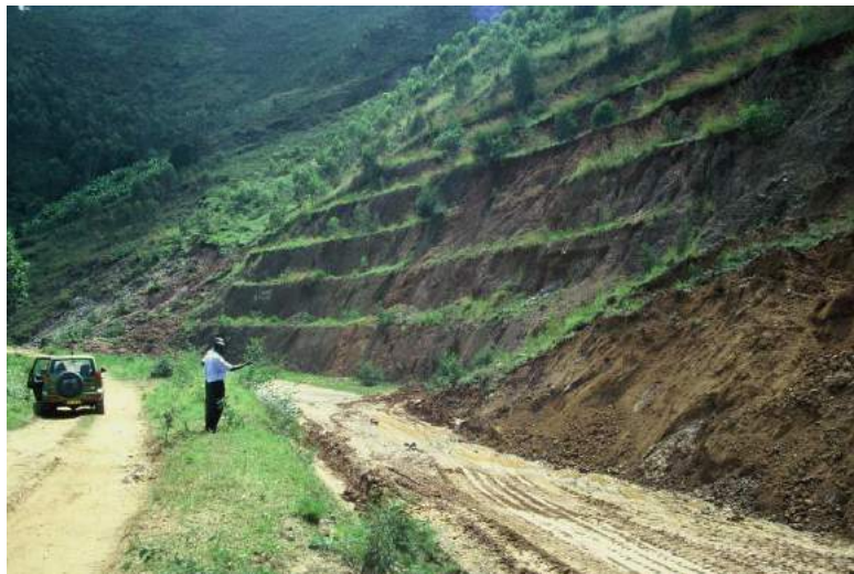
Figure 18: Road closure due to slope failure. Note deviation on the left created to by-pass the failure
