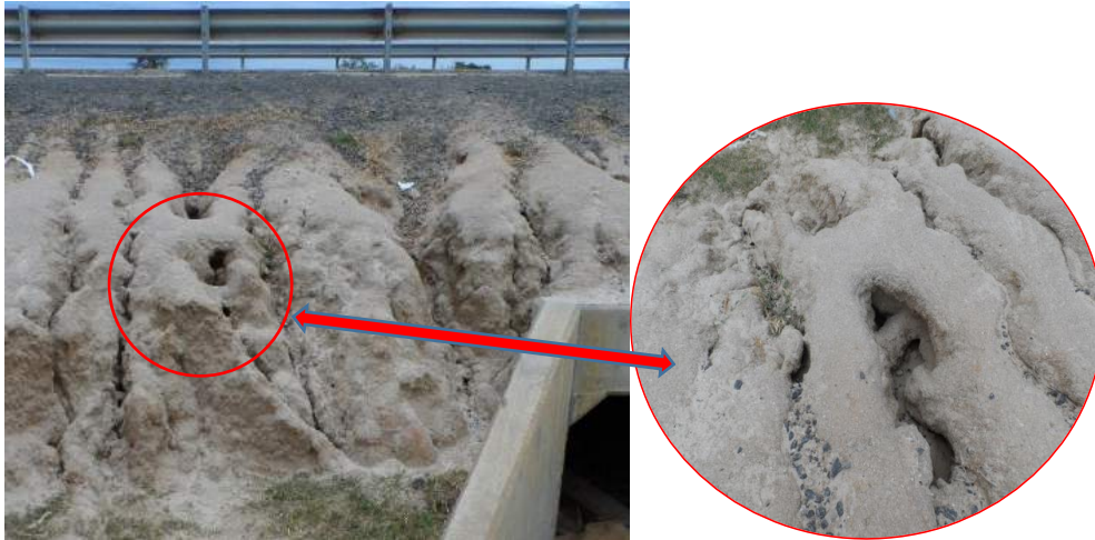
Figure 30: Dispersive soil showing formation of “pipes”
