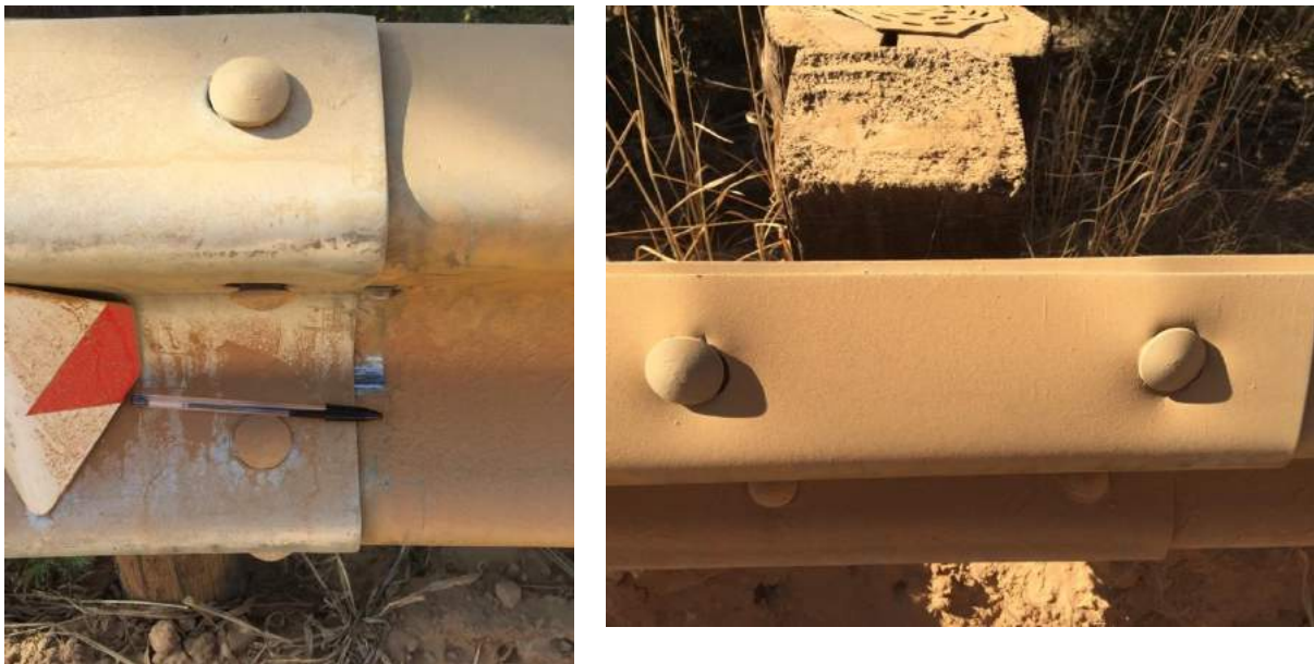
Figure 41: Effect of expansion of metal guard rails: a) loosely tightened and b) tightened so as to avoid thermal movements and cause deformation
