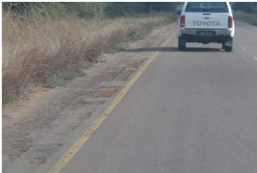
Figure 14: Deterioration of single chip seal shoulder compared with double chip seal on carriage way
