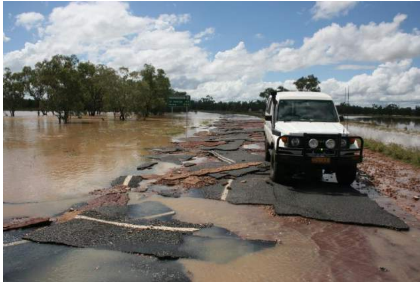
Figure 13: Loss of surfacing caused by high uplift pressures during flooding 2
