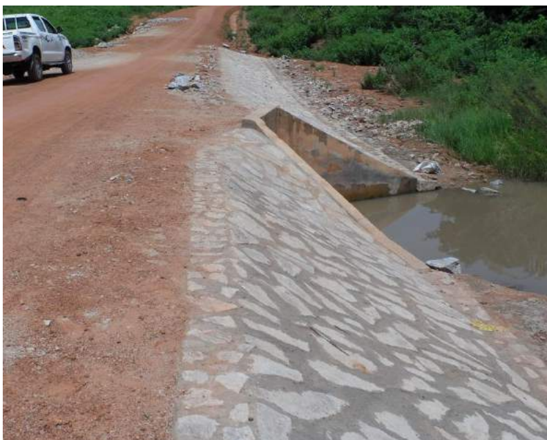
Figure 21: Grouted stone embankment protection of erodible material
