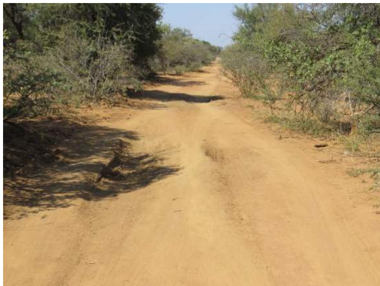
Figure 9: Typical un-engineered earth road showing damage caused by water retention
