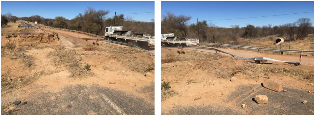
Figure 37: Damage to steel culvert after storm with total loss of embankment. Photograph on right shows final location of metal pipe
