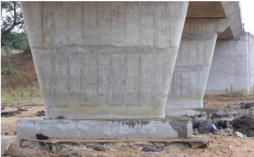
Figure 39: Localised scour around bridge pier footing
