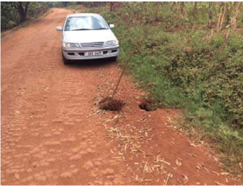
Photo # 08: Damaged culvert entrance, training - Uganda
