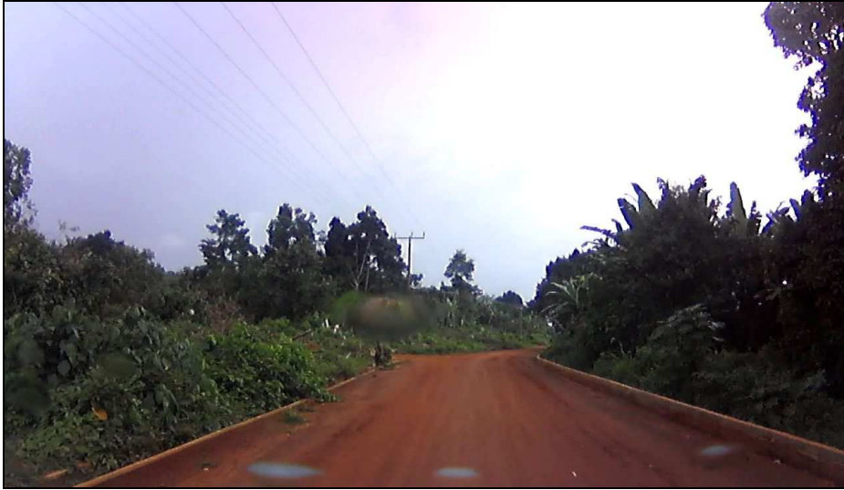
Photograph 3: Section of the Opesika to Samlesi route
