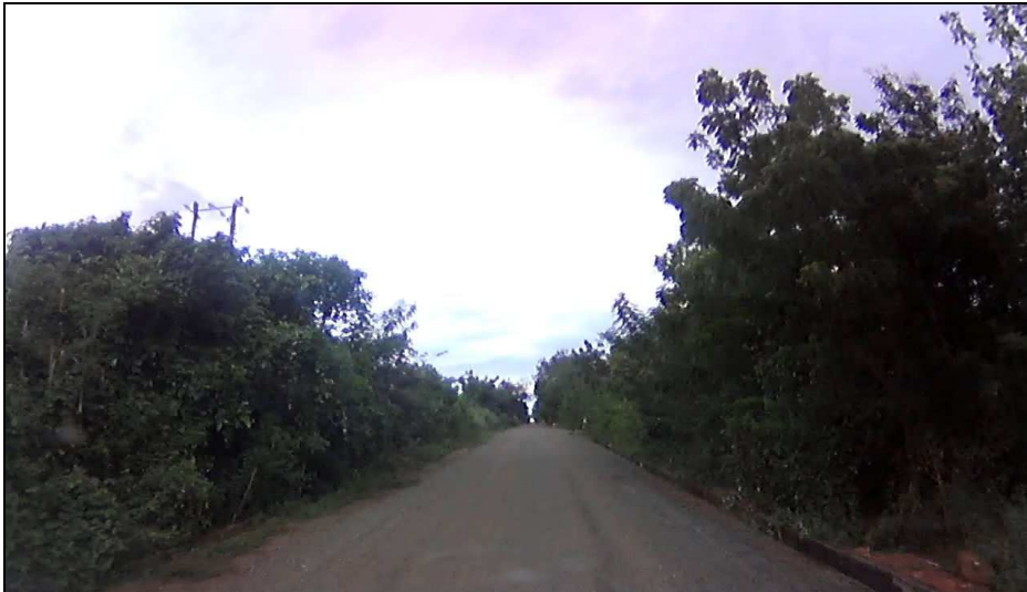
Photograph 4: Section of the Akosombo to Gyakiti route
