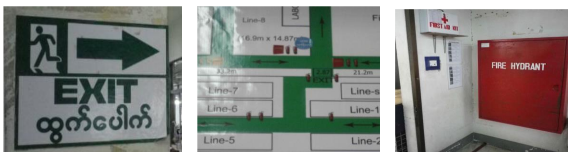
Fig.3 – Fire exit, evacuation route map, and fire hose at a garment factory
