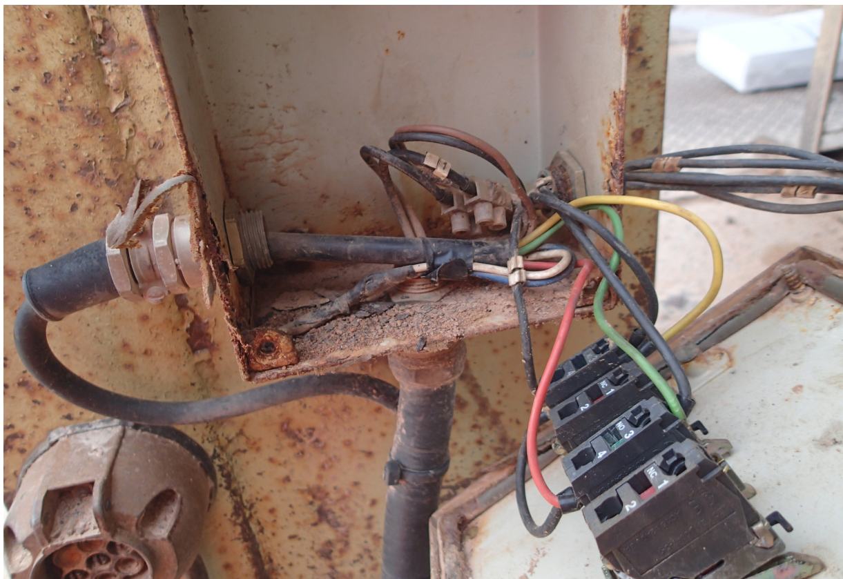
Figure 15: Switch enclosure box on main line side of wagon
