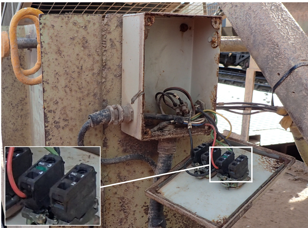
Figure 10: Control panel on mainline side of wagon after the incident
