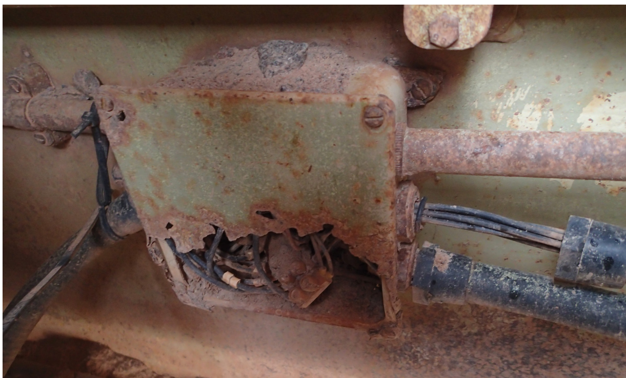
Figure 16: Wiring junction box beneath 'spider' switch
