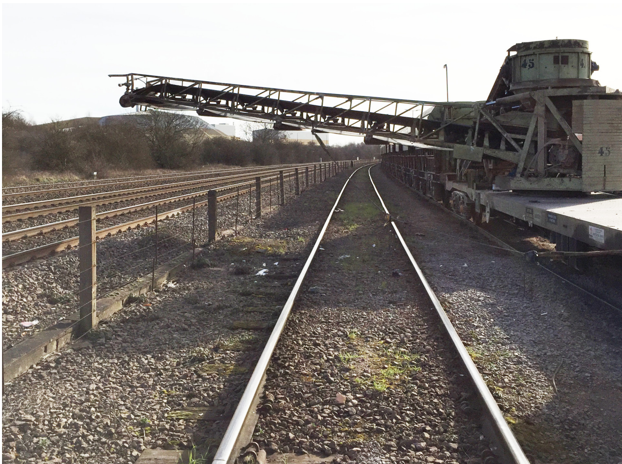
Figure 8: Position of the conveyor boom shortly after the collision (and after a winch had been attached in preparation to move it) (image courtesy of Network Rail)
