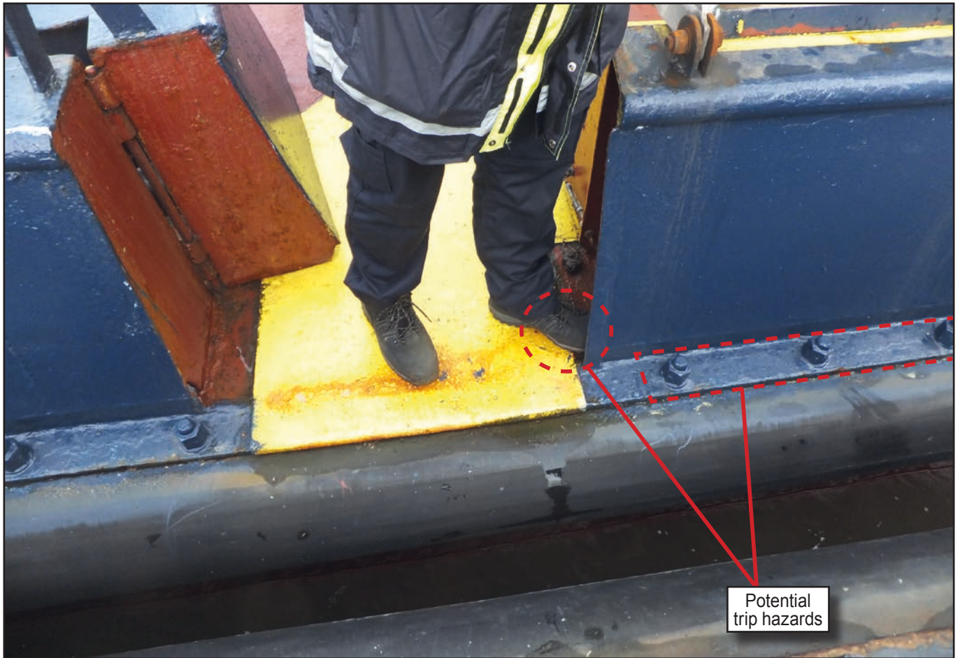
Figure 6: Bulwark structure, fendering and securing bolts
