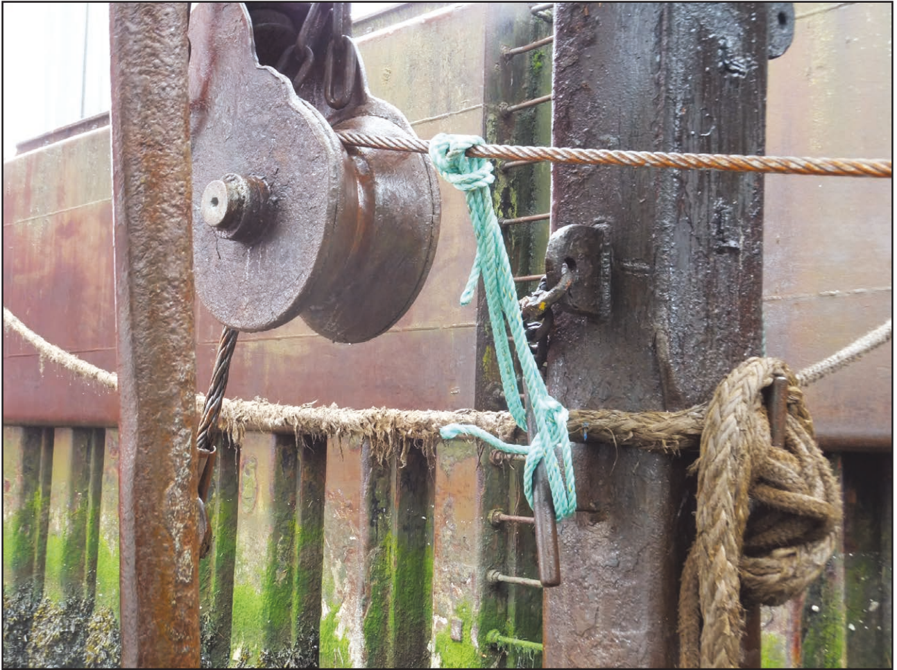
Figure 3a: Reconstruction of rope stopper applied
