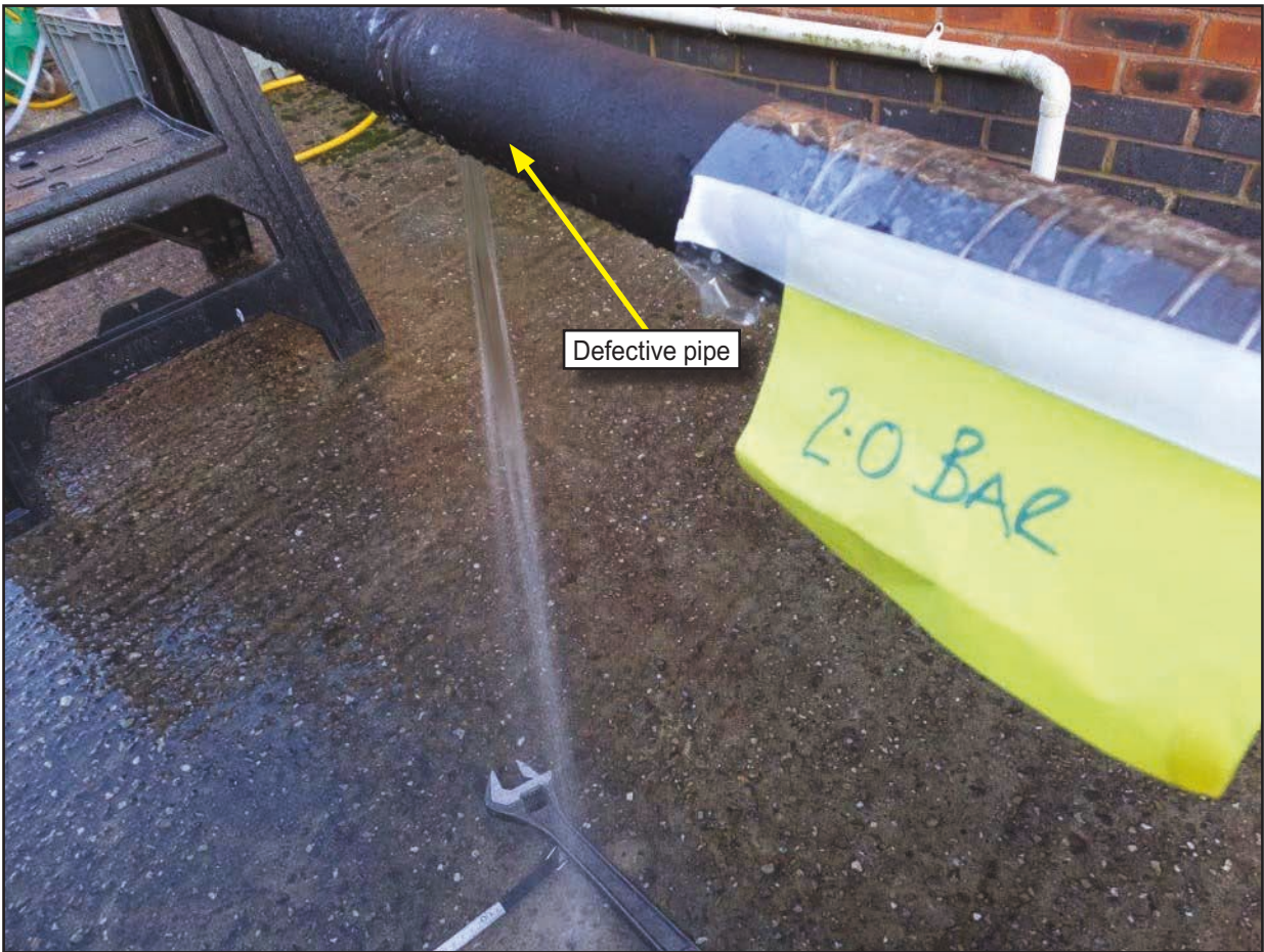
Figure 15a: Spray test
