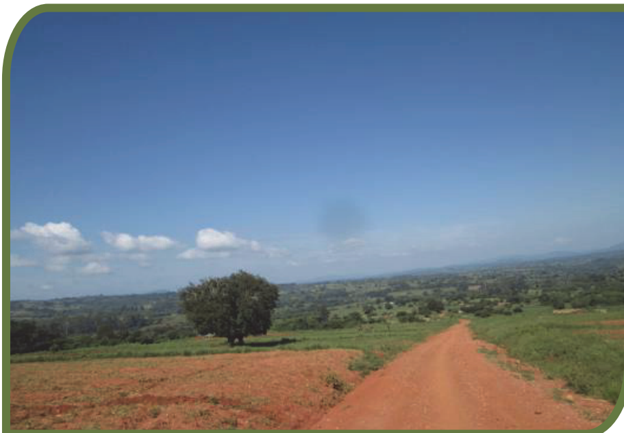
Picture 7: The Ihimbo to Itimbo road
