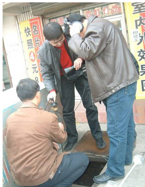
Leak detection in progress
