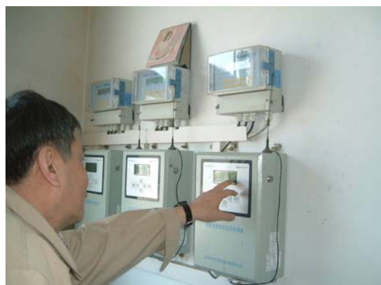
At Beipiao water supply company
